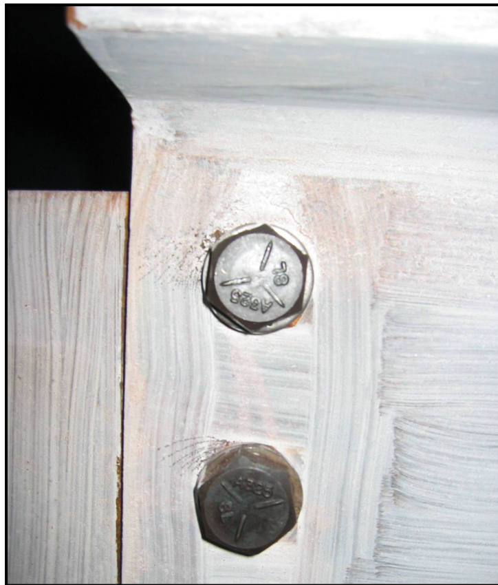
Figure 4.6 Test 7 (7B1C-9-3/8) Yielding in Beam at Bolt Holes
