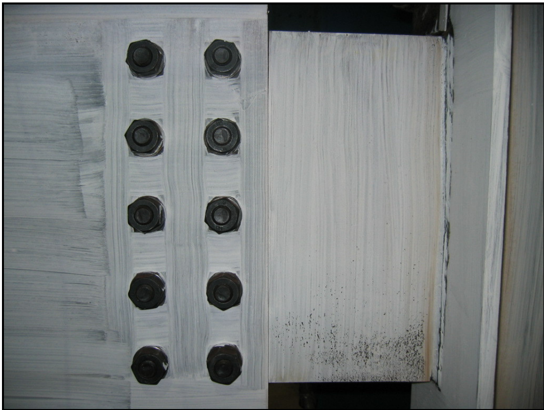
Figure 4.7 Test 8 (10B2C-10.5-1/2) Plate Yielding
