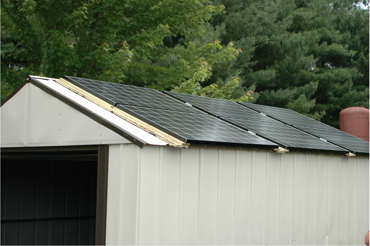
Figure 59. PV Test Building
