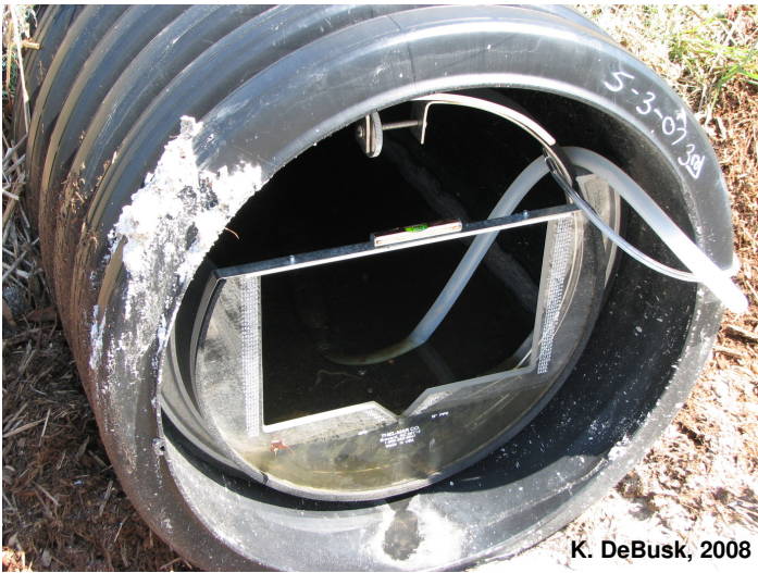
Figure 4.7. Thelmar weir, bubbler level and ISCO intake tube installed in the inflow pipe of the bioretention cell.
