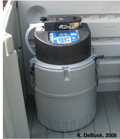
Figure 4.8. ISCO 6700 sampler installer at the inflow pipe of the infiltration trench.
