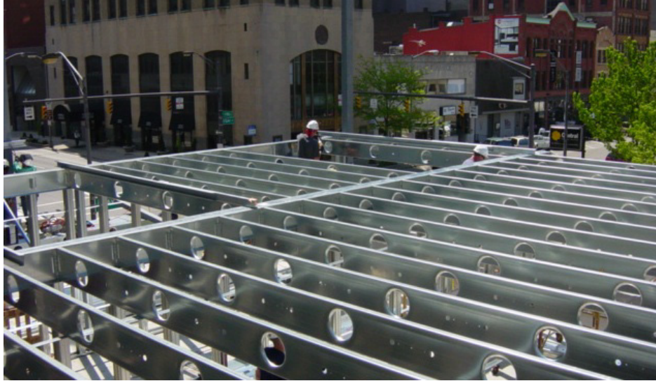
Figure 1.5 Cold-formed steel framing with edge-stiffened holes
