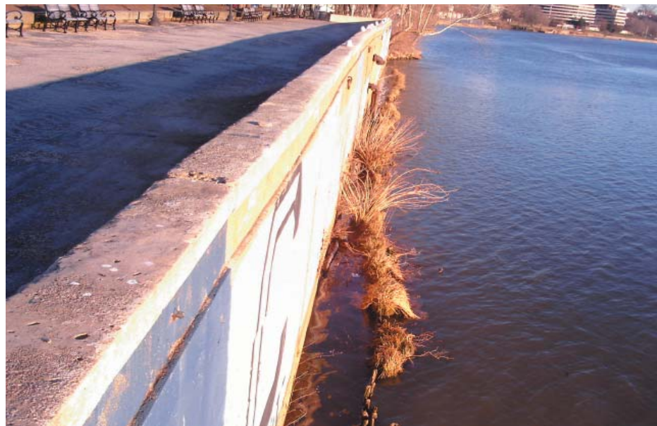
Figure 5.2. The floodwall distances people from the river.
