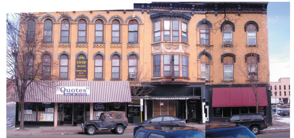
Figure 6.3. Janesville’s typical downtown historic structures have small local shops with residences above.
