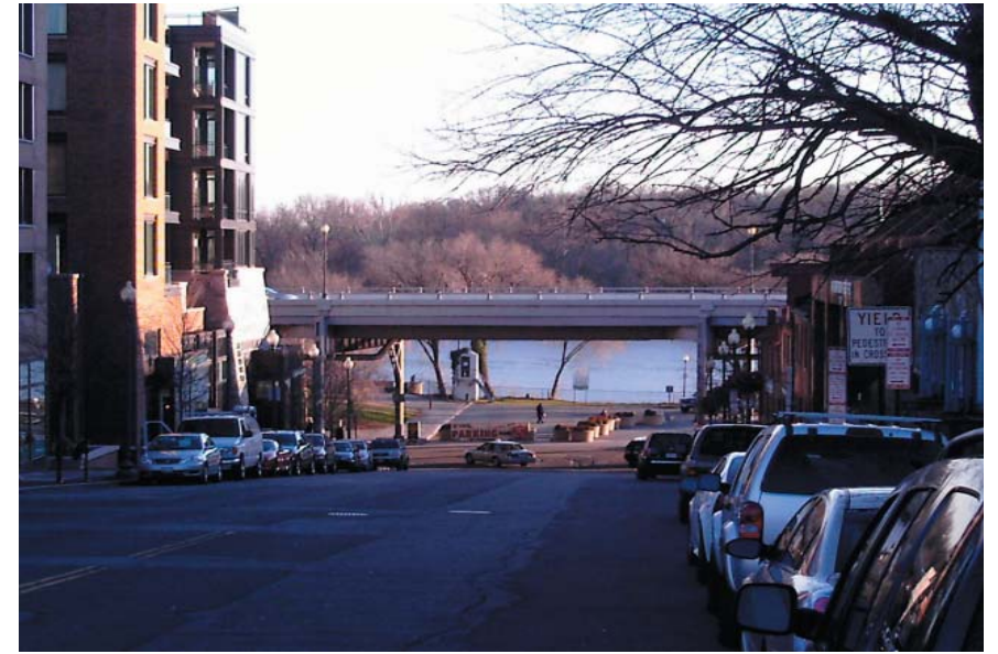
Figure 4.28. The Whitehurst Freeway blocks views from perpendicular roads to the river.
