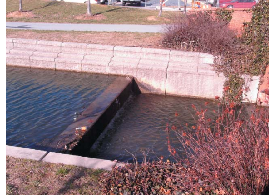
Figure 4.13. This small dam creates a sound that can be heard nearby.
