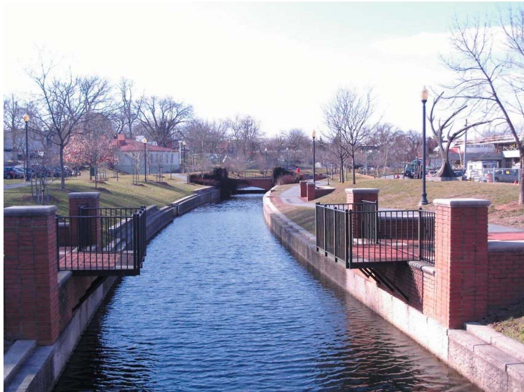
Figure 4.11. Carroll Creek is a concrete lined channel.
