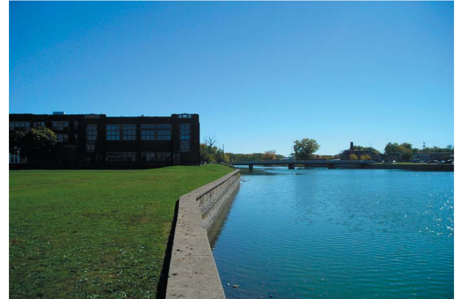
Figure 6.4. Janesville is protected from the Rock River by a floodwall that spans the entire downtown.
