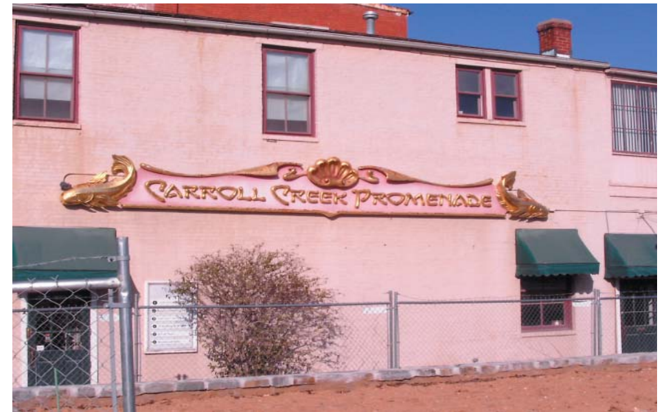
Figure 5.3. The building's architecture does not focus on water.
