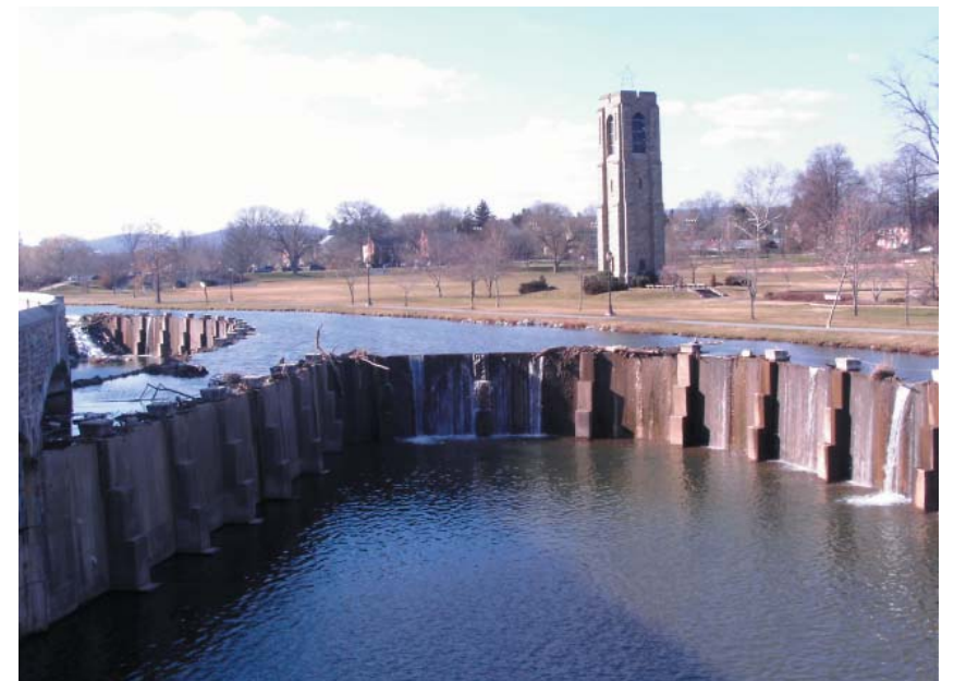
Figure 4.14. The above ground creek on the left goes downtown while floodwaters fall to the basin below and into underground culverts.
