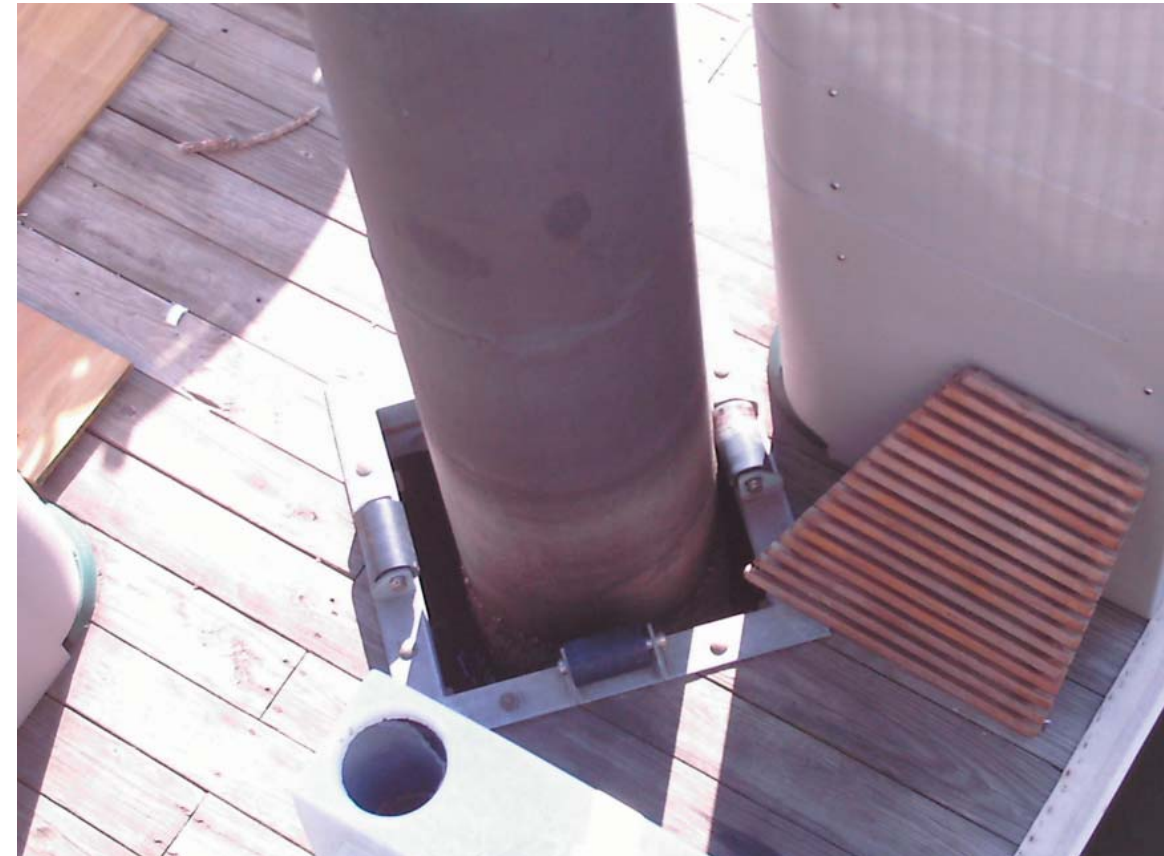
Figure 4.3. The dock is anchored by poles, so it can move vertically.
