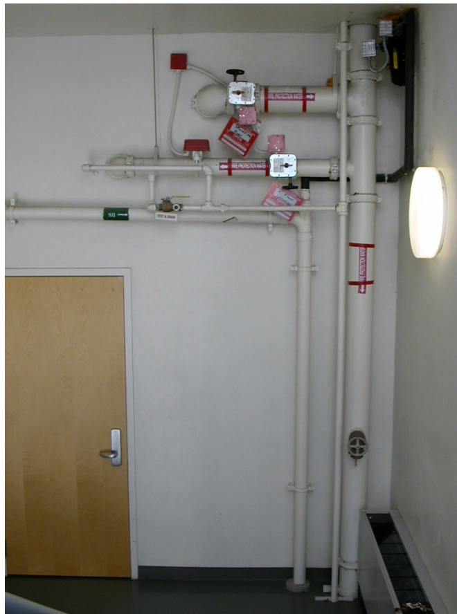
Figure 6.4: Fire Standpipe Riser
