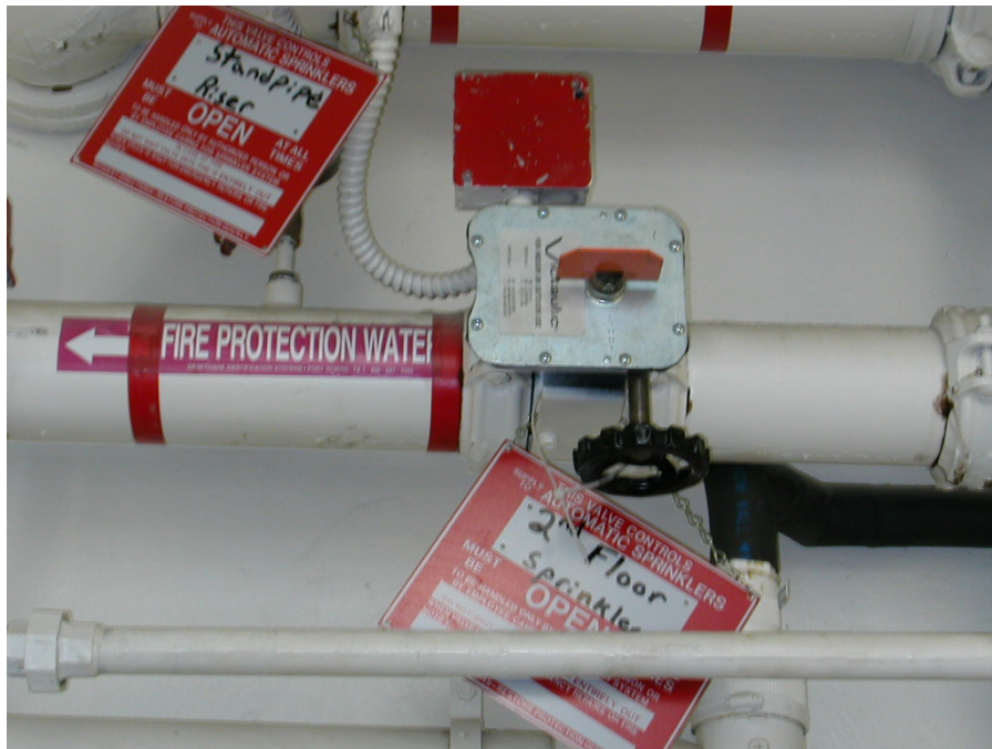
Figure 6.6: Durham Hall Combined Sprinkler/Standpipe System
