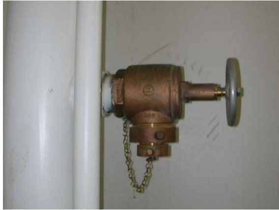
Figure 6.5: Hose Connection Valve
