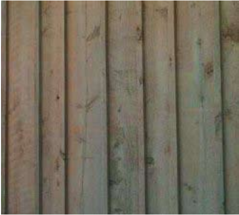
Cypress siding for the exterior
