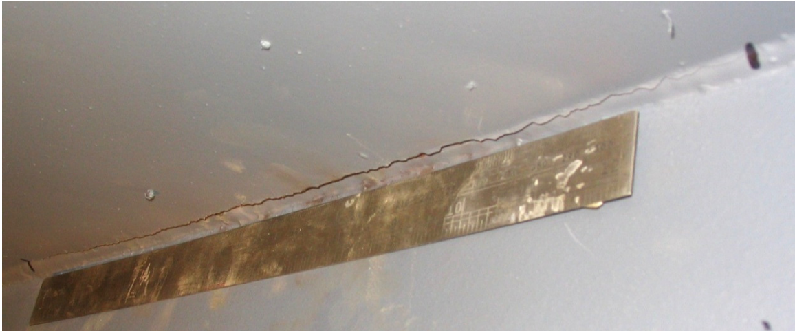
(a) Before repair
