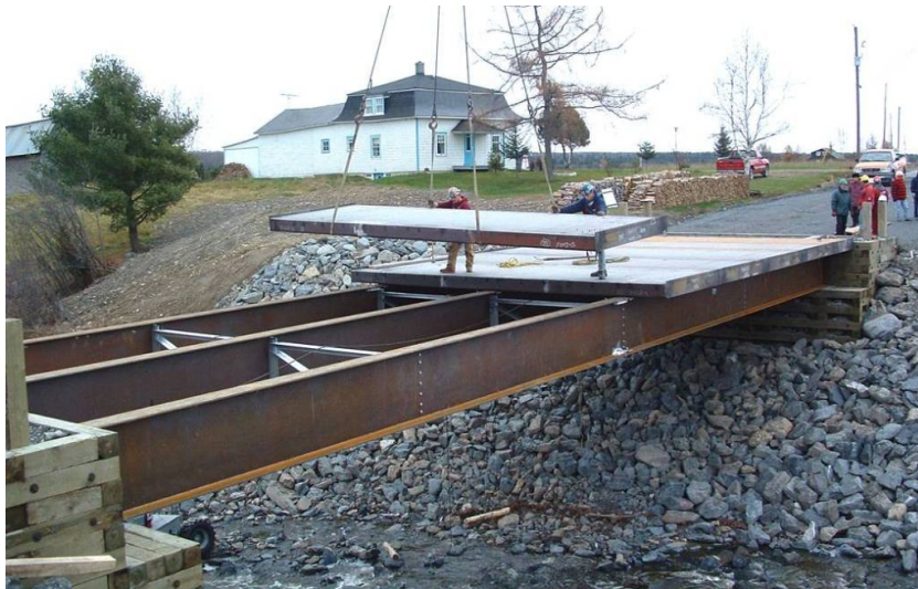
Figure 2.3: Shenley Bridge deck installation
