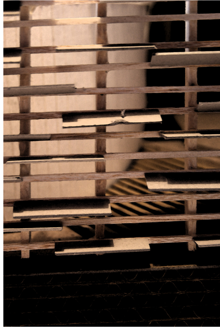
cafe stair beyond copper fin facade
