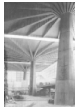
International Labor Exposition Hall, Turin, Italy, Pier Luigi Nervi (1961). The concrete column tapers 18 to 9 feet in an 82 foot run.
