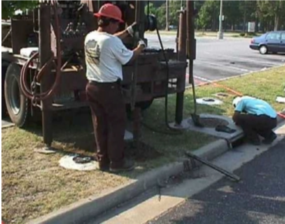
Photograph 1. Borehole advanced in the immediate vicinity of well MLS-12 utilizing hollow-stem auger drilling equipment and split-barrel samplers.
