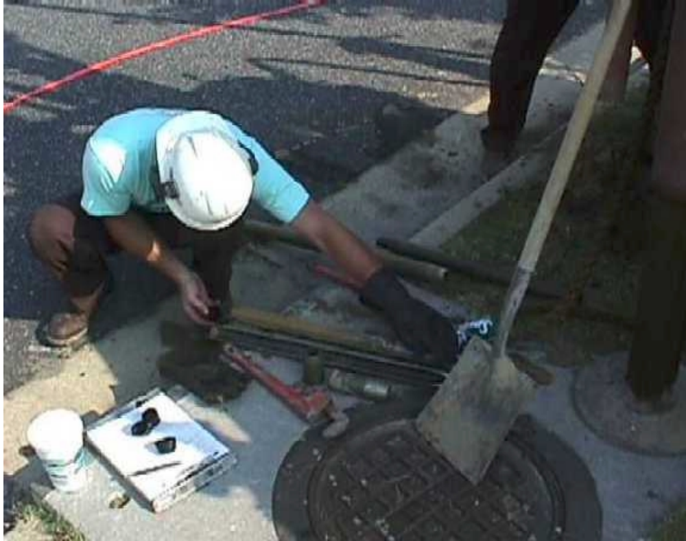
Photograph 2. Aquifer sediments retrieved from 2.5 to 3.5 m below ground surface in sterile acetate liners. Driller is capping liners.
