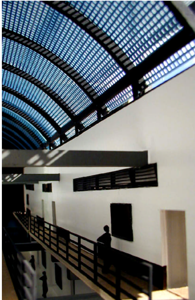
Ventilation louvers in Atrium
