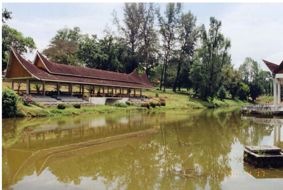
Figure 4. Park's amphitheatre which has deteriorated
