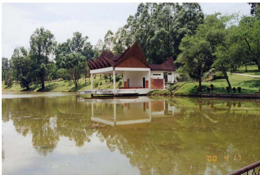
Figure 5. Park's stage which has deteriorated
