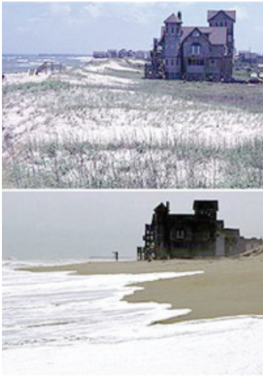
Fig. 2.4: Erosion along the Outer Banks, 1999 (top) and 2004 (bottom). (source: © Gary Braasch)
