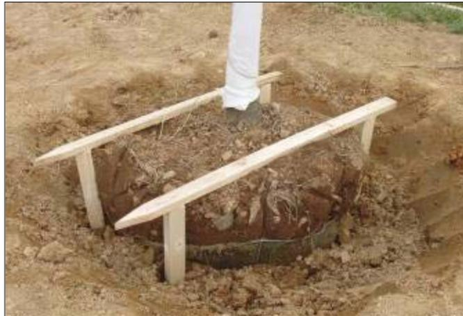
**Figure 2.1** – Generic root ball anchoring system consisting of four vertical anchors and two horizontal crosspieces.
