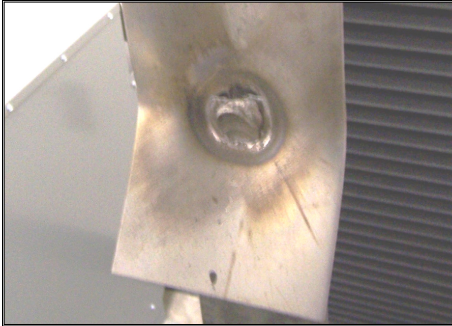
Figure 3-5: Sheet Tear Failure
