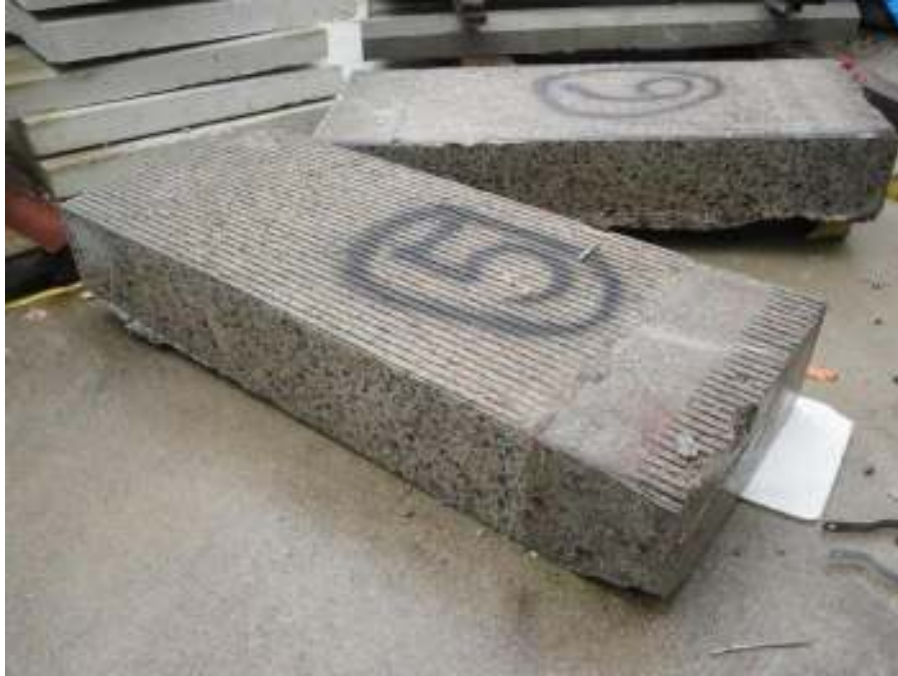
Figure 3-1. Typical Specimens Cut From the I-81 Bridge Deck
