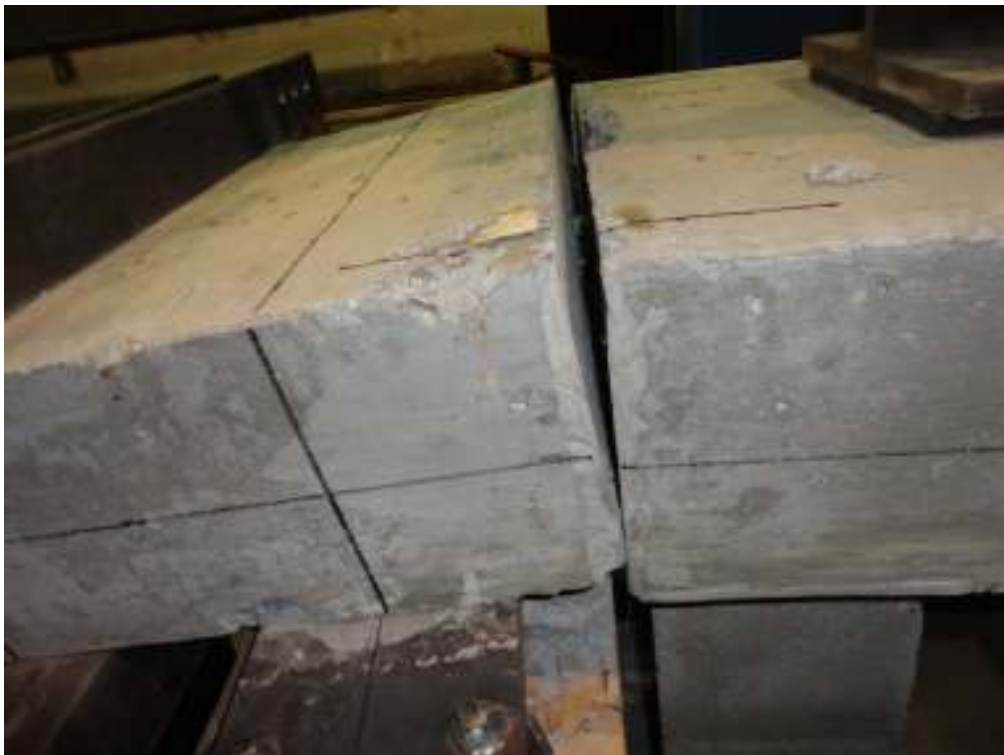
Figure 5-29. Opened Joint after Fatigue Failure, Closure Pour Section on Right Side
