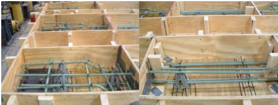
Figure 3-3. Formwork of Cast Slabs with Reinforcing Steel in Place
