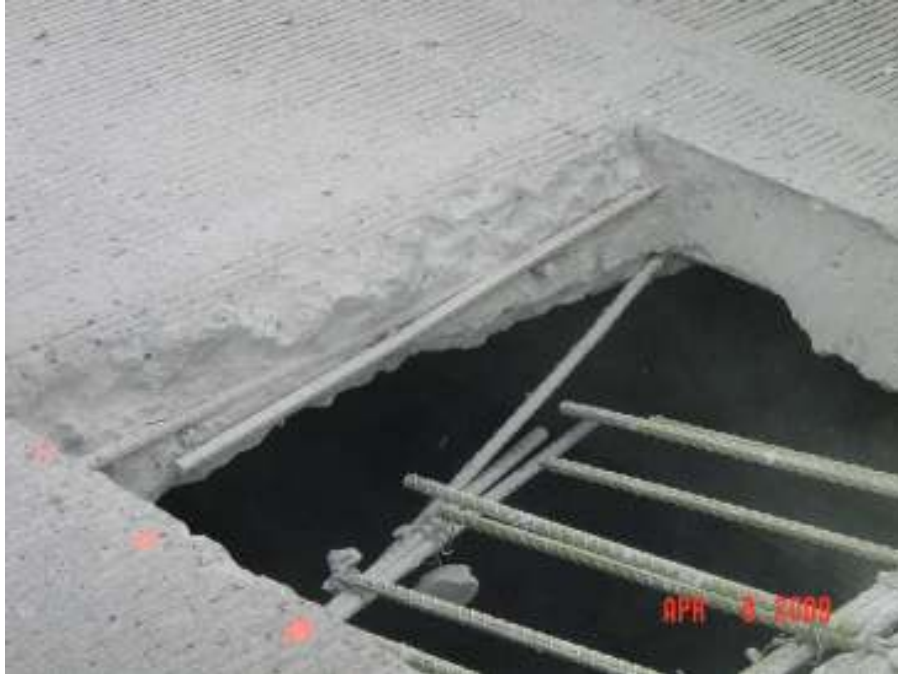
Figure 1-1. Failed Closure Pour Section (Sprinkel, et al., 2010)
