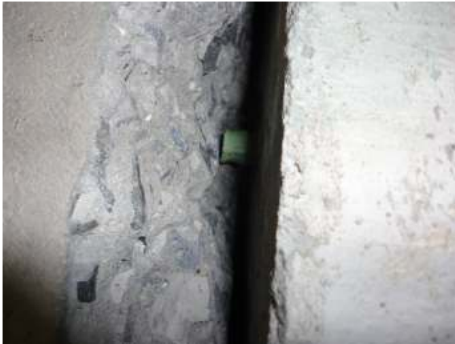
Figure D-14. Top View of Failed Rebar at Joint 2 (Spalled Concrete Removed)
