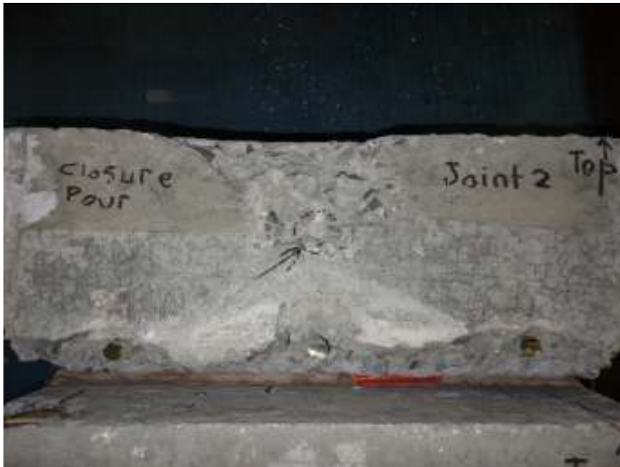
Figure D-18. Closure Pour Face of Joint 2 with Failed Top Rebar
