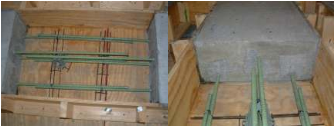
Figure 3-5. Closure Pour Section Prior to Second Concrete Placement
