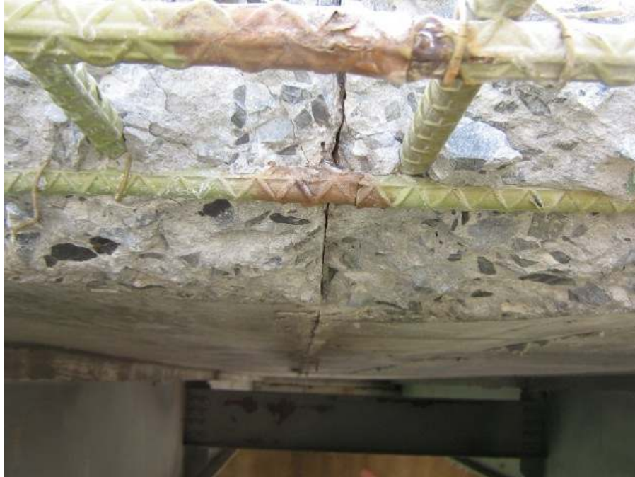
Figure 1-2. Sheared Bars at Closure Pour with Corrosion Damage (Sprinkel, et al., 2010)
