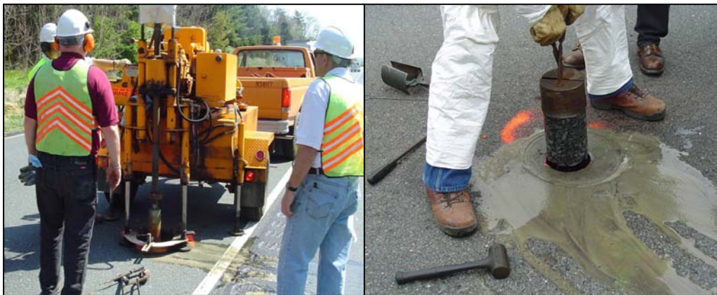
Figure 4. Coring Machine and Core Extraction
