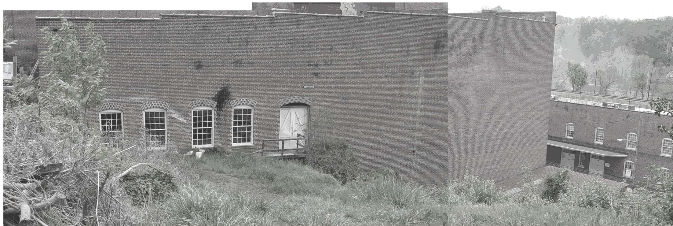
Western facade of building: 3rd Floor (retail entrance)
