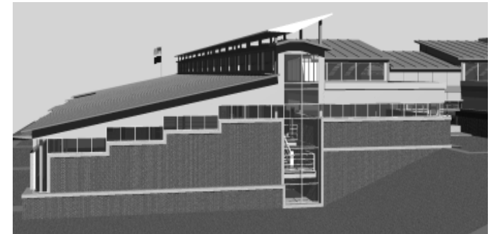
PUBLIC AREA MAIN STREET ELEVATION SHOWING WIND FIN AT CLERESTORY
