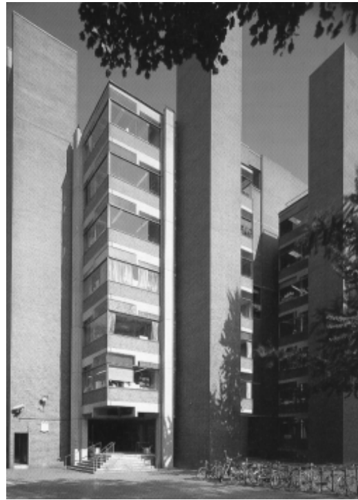
Louis I. Kahn Richards Medical Research Building, University of Pennsylvania Philadelphia, Pennsylvania, 1957-1965
