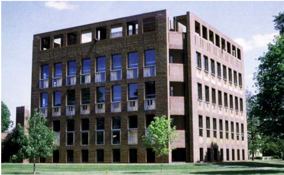
Exterior of Louis Kahn's Library at Phillips Exeter Academy (2)
