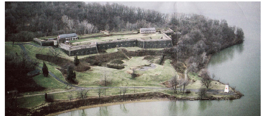
Figure 18. Fort Washington, MD. (Interior).
