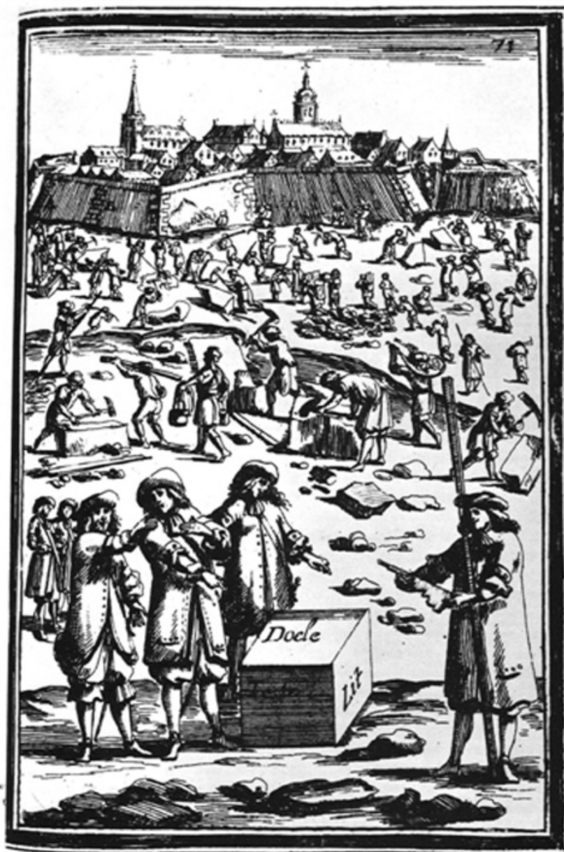
Figure 13. Stone-cutting materials for construction of fortification (Duffy).
