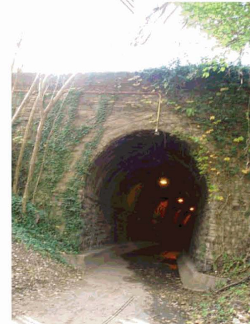
fig. 7.3 Photograph of tunnel
