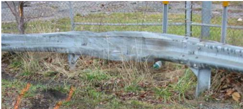
Figure 133: An example of w-beam guardrail that has been flattened by an impact from a large van.
