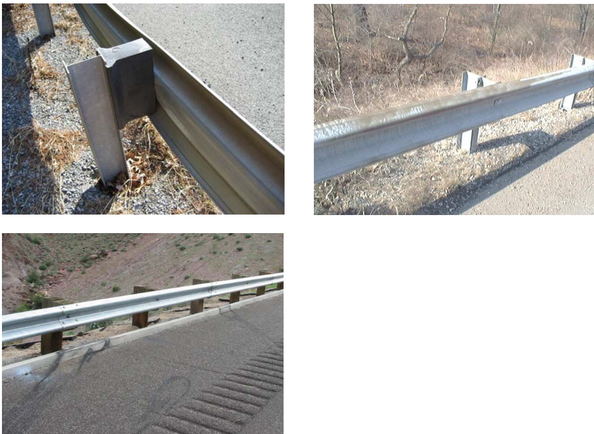
Figure 1: Examples of various types of strong-post w-beam guardrail systems. Steel post with plastic blockouts (top left), steel post with steel blockouts (top right), wood post and blockout (bottom left).
