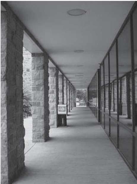
Left: Once on the level of Burchard Plaza the minor axis moves down the loggia formed by the east facade of GBJ. Moving further into campus this covered walkway expedites the passage to the Drill Field. (Photo by author)
