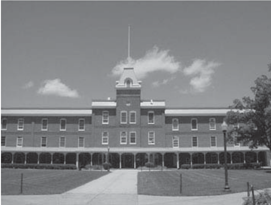
Barracks No. 1 (Lane Hall), present day. The central building of the Upper Quad, this structure served as the focal point of campus expansion during the first fifty years of Virginia Tech. (Photo by author)
