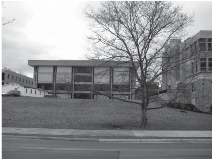
A view through the gap between Cowgill Hall and Bishop-Favrao Hall to GBJ in the background. This photo shows the use of concrete in the new building to connect with the context of its neighbors.(Photo by author)
