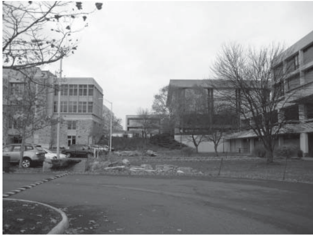
With Bishop-Favrao Hall completed, the only connection to the plaza between Derring and Cowgill, or to the steps leading up to GBJ, is a set of concrete stairs tucked into the corner of the retaining wall at Derring Hall. (Photo by author)
