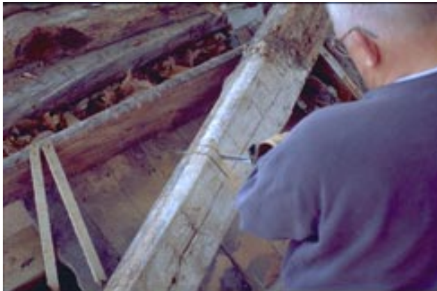
Fig. 33 Photograph showing thickness of sample taken from a floor joist.
