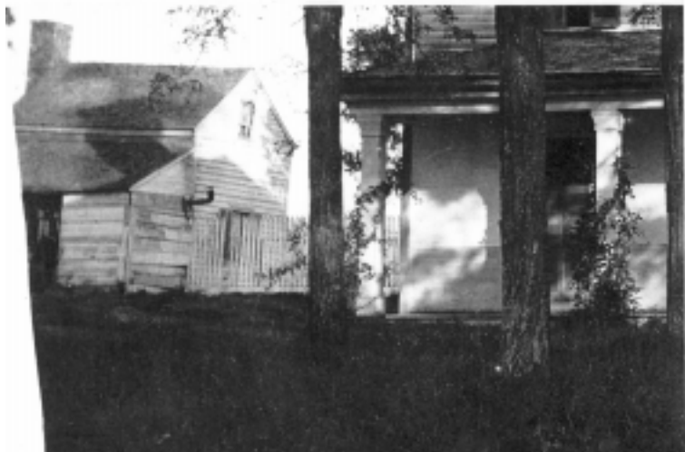
Fig. 10 Close-up of outbuilding that probably served as a servant's cabin. From a photograph hand-labeled "professor's house, 'Solitude' 189-," in reference to the main house. Newman Library Special Collections
