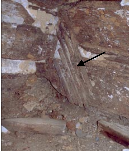
Fig. 20 1999 photograph showing some of the surviving original lath, nailed directly into the wall logs (NE corner of log pen). Some whitewash can be seen on the logs also.
