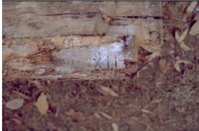
Fig. 38 Log floor joist bearing carpenter's mark.
