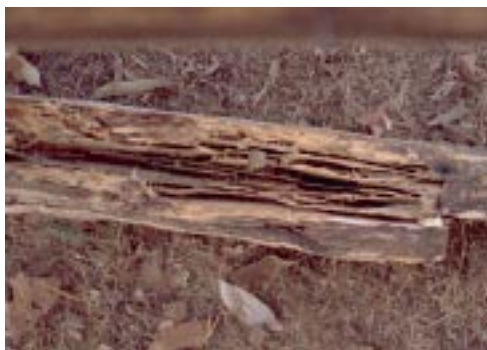
Fig. 26 Termite damaged log floor joist
