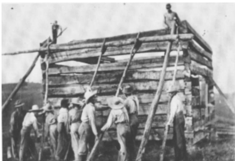
Fig. 18 Late 19 th century photograph showing how log pens similar to the one at Solitude were typically constructed. Each log was pushed up on skids, using long poles. Notice that a window has already been cut so the builders could enter the pen's interior. Notice also the large gaps caused by bowed logs. Hutslar, Donald A. Log Construction in the Ohio Country, 1750-1850 . (Athens: University of Ohio Press, 1992), frontispiece.
