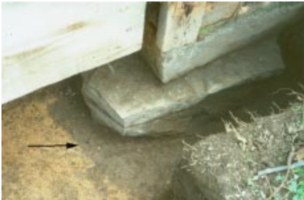
Fig. 17 Edge of hole dug for footer placement is clearly defined by difference in soil color.
