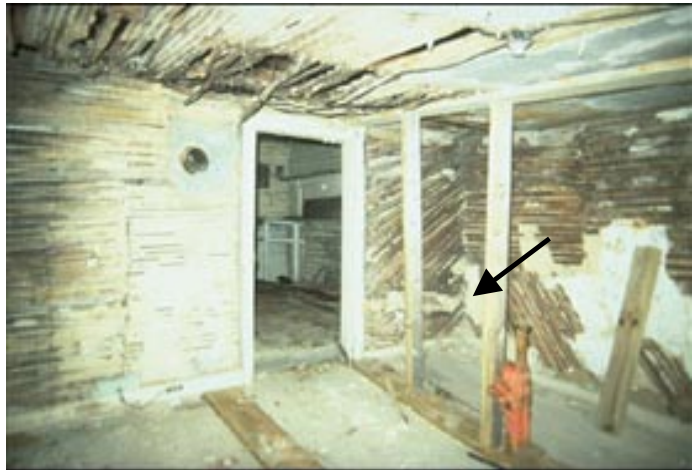
Fig. 21 1989 photo of lower floor of original log section, looking into the frame addition through the doorway. Note the severe loss of plaster. Arrow points to the same corner as the arrow in Figure 20.
