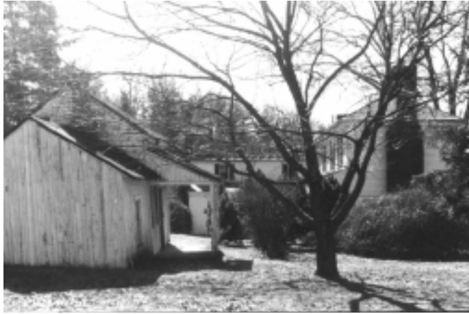
Fig. 11 1989 photo of outbuilding and main house from the north side.
