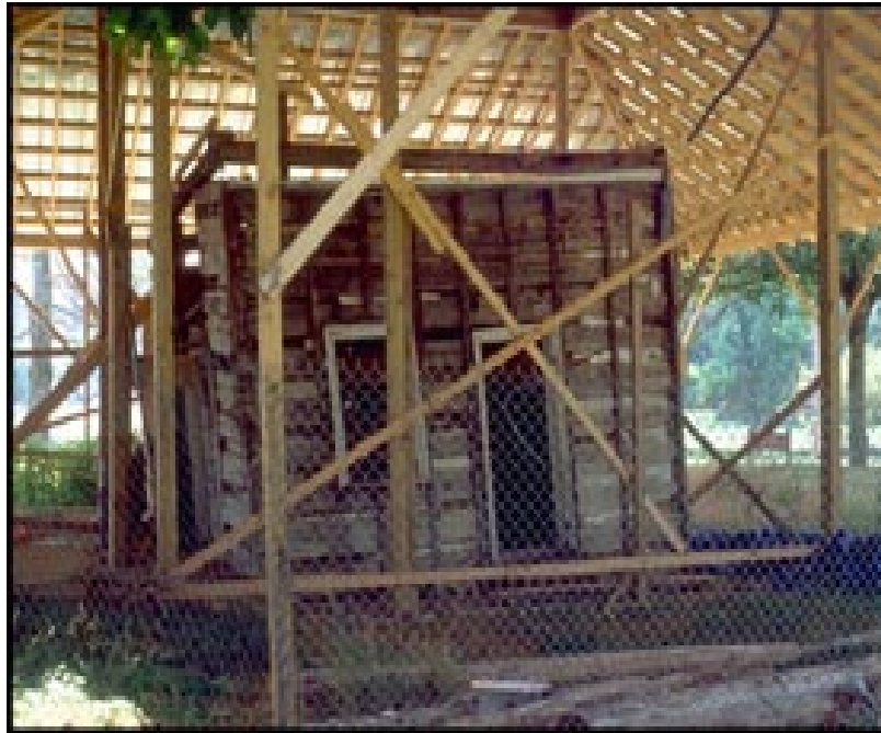
Fig. 4 September 1999 photograph of outbuilding under its extravagant new shelter. Note the substantial bracing (left, background) now required to prevent further slumping.
