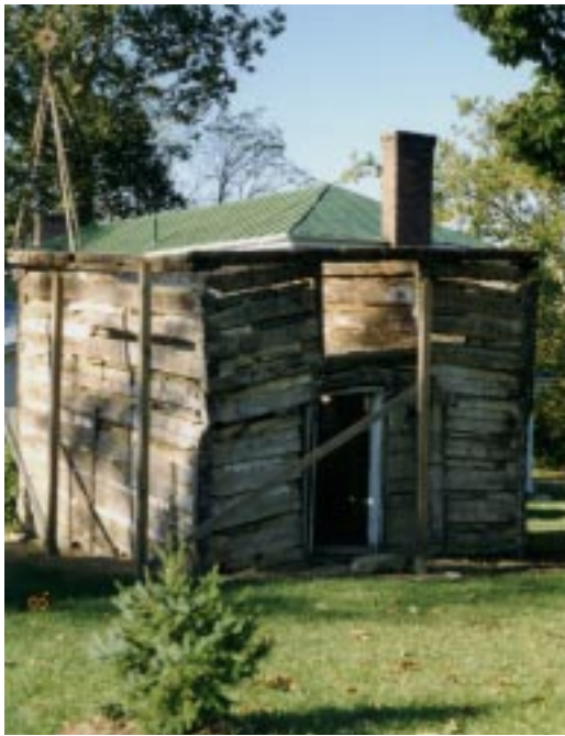
Fig. 13 1998 photograph of slumping outbuilding (servant's cabin) remains.
