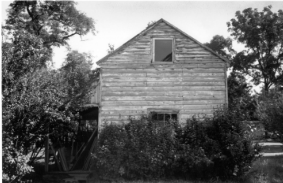
Fig. 1 View of the outbuilding from the south, photo taken in the late 1970s or early 1980s.
