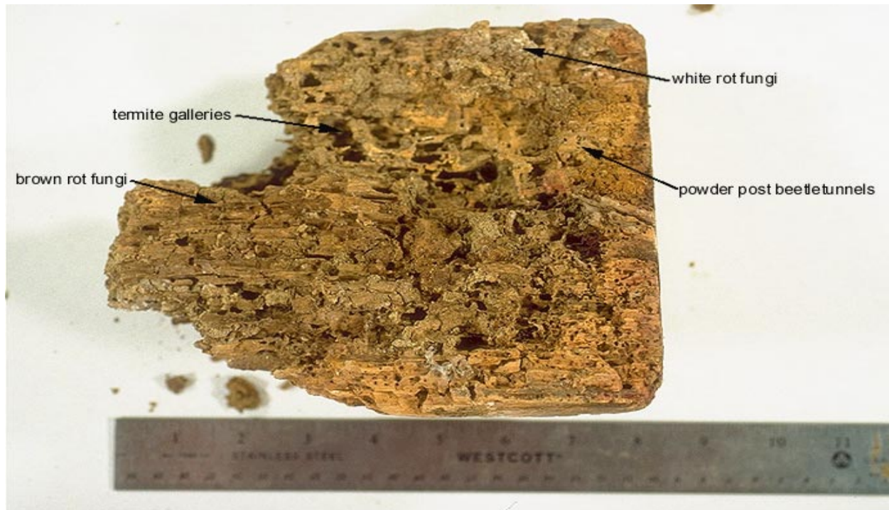
Fig. 31 Severely deteriorated lower course wall log (not included in Table 1).
