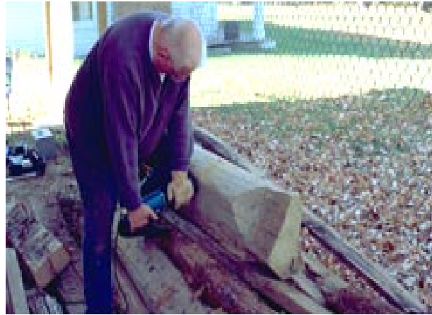
Fig. 32 Dr. Heikkenen saws a sample from log sill. The sill had already been replaced due to its badly deteriorated condition.
