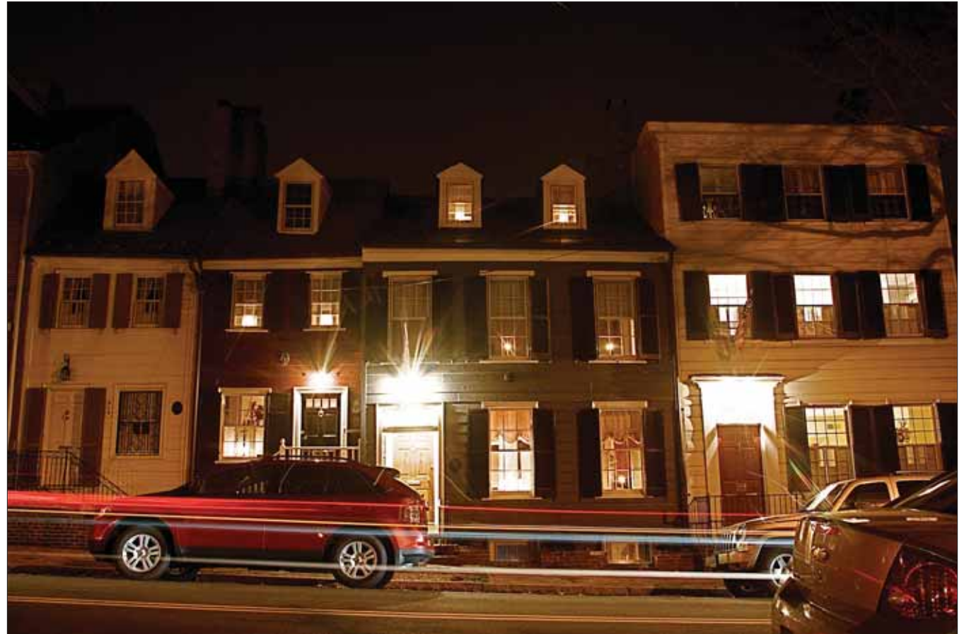
Time Passing @ Typical Neighborhood Row House on Prince Street Alexandria, Virginia
