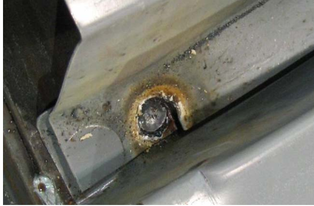
Figure 4-8: Weld Crack from Diaphragm Loading
