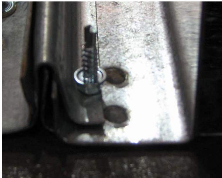
Figure 4-7: Side-lap Detail
