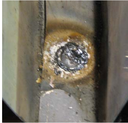
Figure 4-6: Puddle Weld
