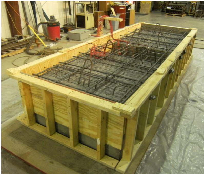
Figure 49: Formwork for CIP Deck Concrete
