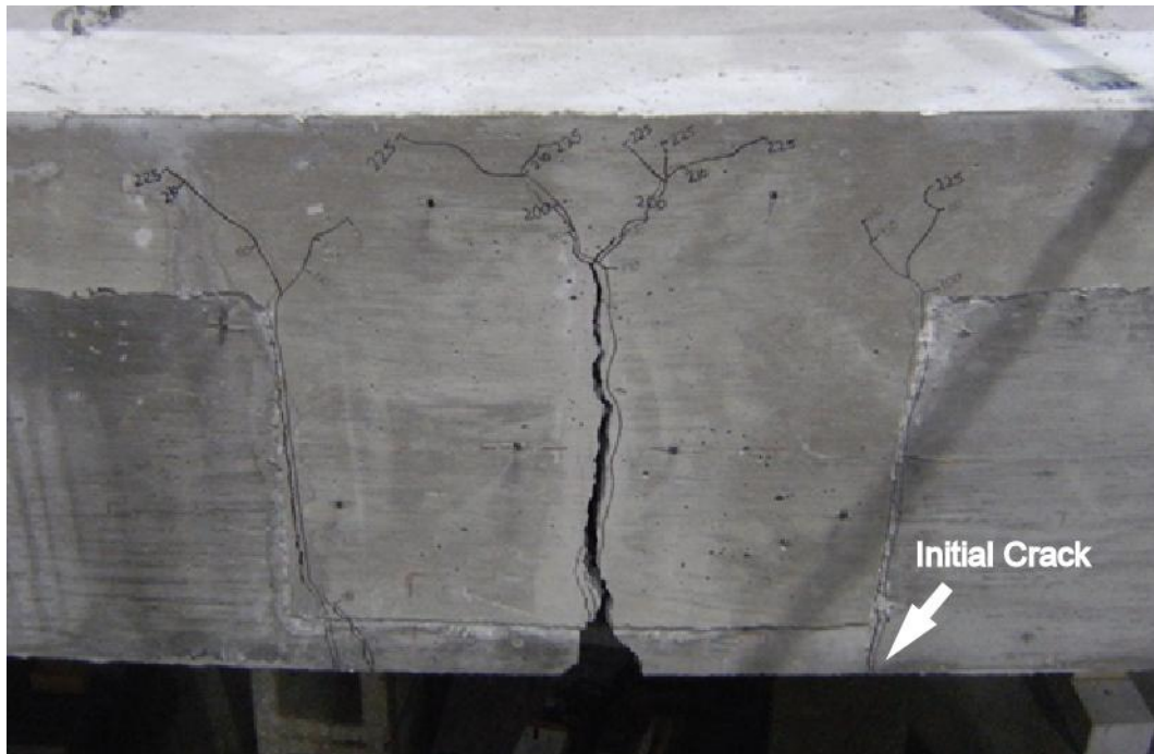
Figure 59: Cracks on Embedded Plate Inverted-T Specimen (photo)
