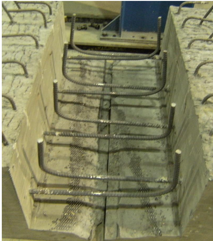
Figure 45: Poor Roughened Surface and Flanges
