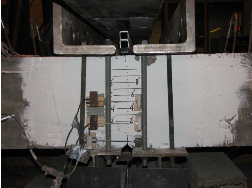
Figure 8: Clamping System Used to Provide Rotational Restraint (Courtesy of Mn/DOT)
