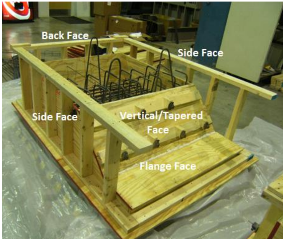
Figure 42: Formwork, Pencil Rod, and Rebar
