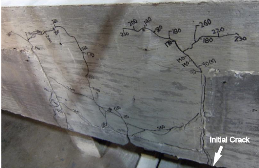
Figure 58: Cracks on Extended Bar Specimen (photo)
