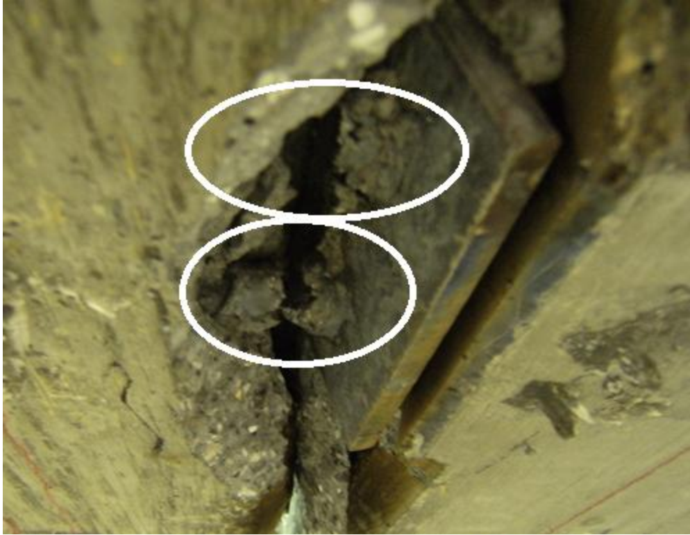
Figure 92: Embedded Plate Inverted-T Connection Failure (photo)
