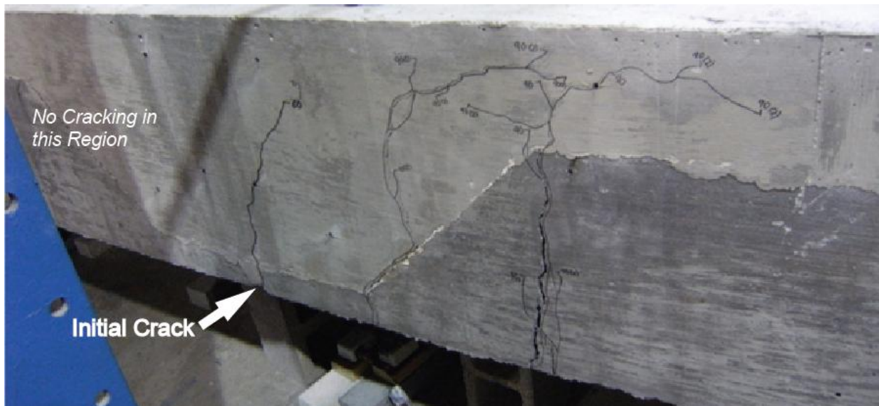
Figure 61: Cracks on No Connection Specimen (photo)
