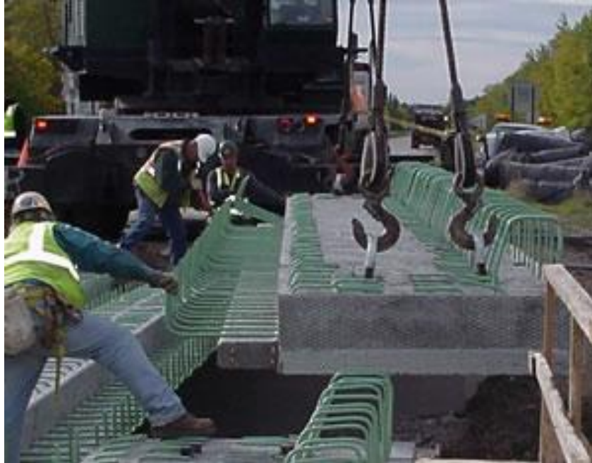
Figure 13: Workers Installing Inverted-T with Extended Bars Into Position (Gonzalez)
