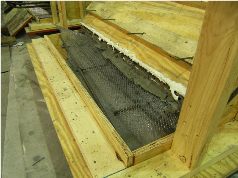
Figure 44: Flange of First Girder Placement (Photo)
