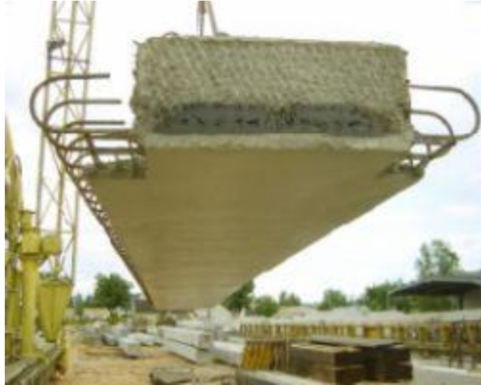
Figure 3: Poutre-Dalle Precast Girder from France (Courtesy of Federal Highway Administration)
