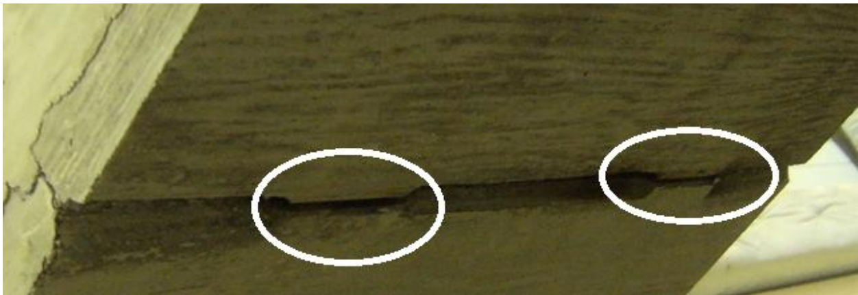
Figure 87: Plates Exposed to Elements
