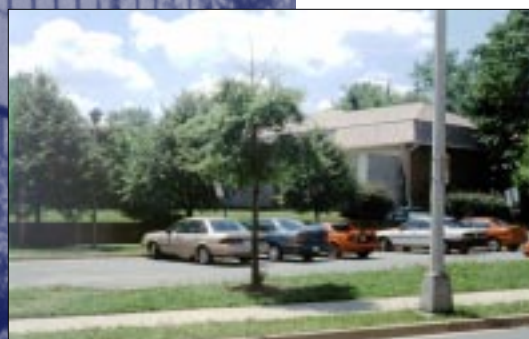
Conflict of interest in a residential neighborhood?: VEPCO transformer yard on Monroe Street.
