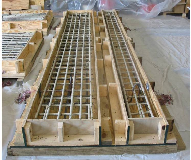
Figure 3.1 - Construction of 1 ft and 2 ft decks
