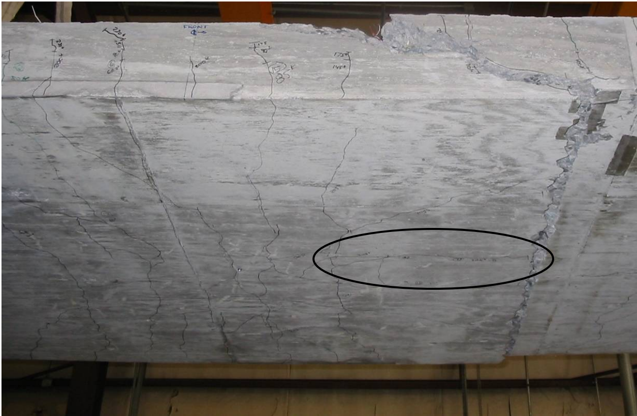
Figure 4.28 - Cracking of the underside of the 5 ft shear specimen. Note the circled crack extending towards the location of the center support.
