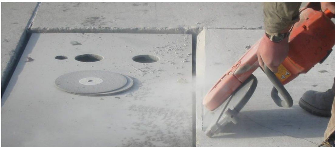
Figure 3.16 - Chamfering the forward edge of the weigh station specimen
