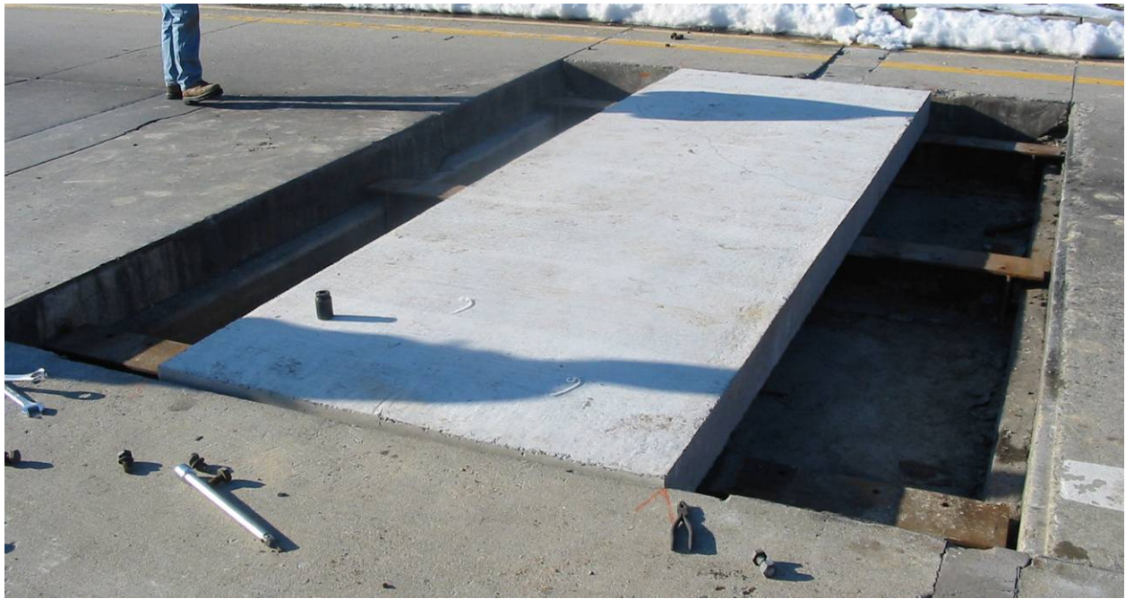
Figure 3.13 - Installation of weigh station specimen on 12/10/2002
