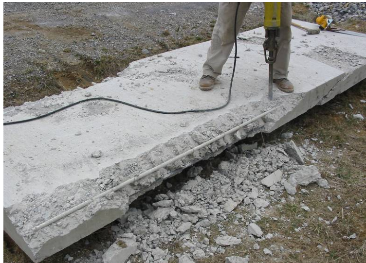
Figure 3.19 - Extraction of GFRP rebar
