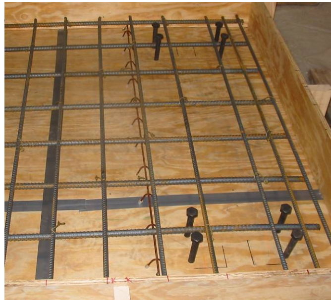
Figure 3.2 - Bottom mat bar spacing
