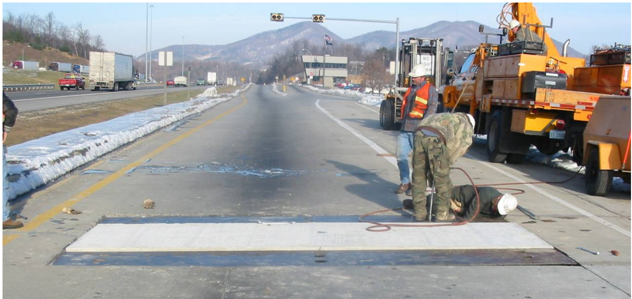
Figure 3.14 - Installation of weigh station specimen on 12/10/2002.
