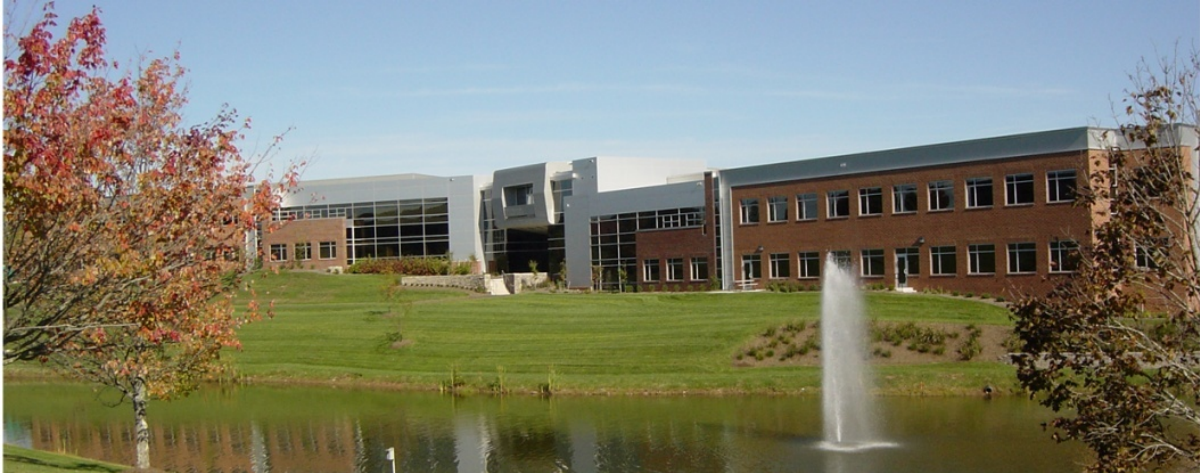
Figure 1.8 - Water pond, a part of the geothermal heat pump system (photograph by Kongkun Charoenvisal, 2007).
