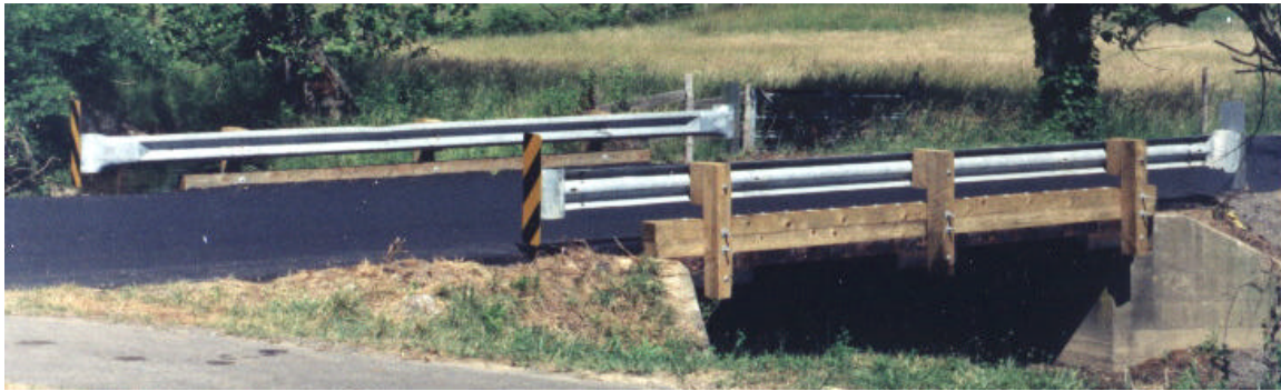
Figure 1- 1: Rehabilitated Tom's Creek Bridge
