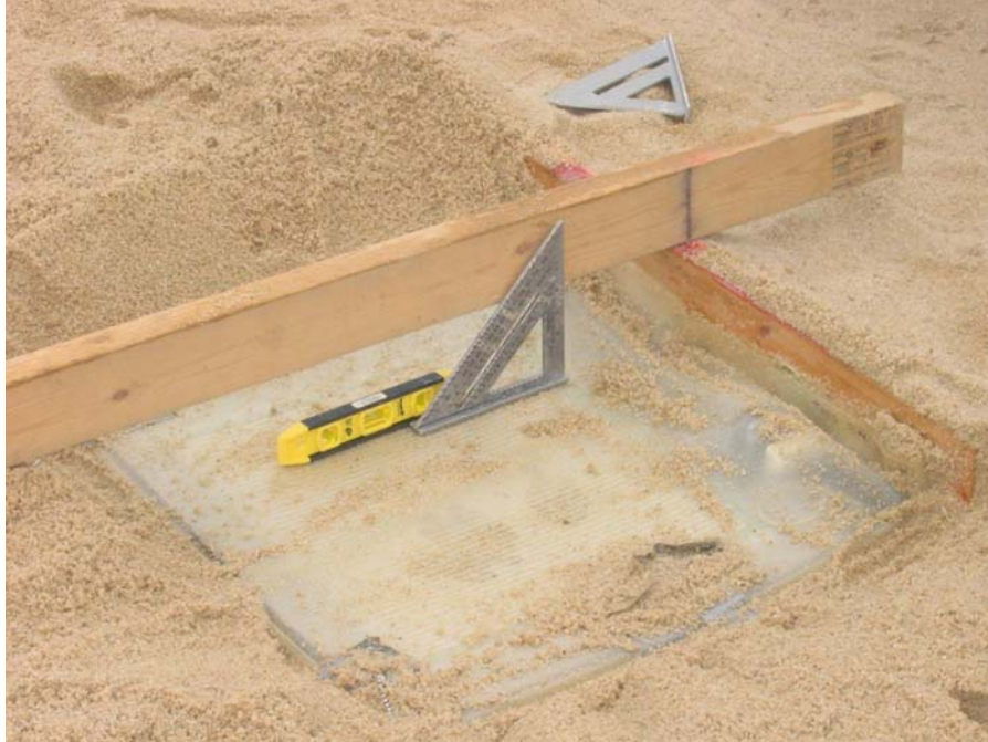
Figure 6-12: Pressure Sensor Burial Using Level and Measured Height to Top of Sand (Used in Spring/Summer 2007 Tests)
