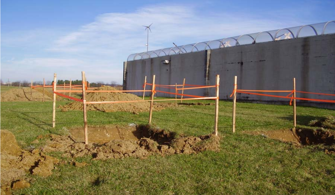
Figure 6-5: Winter 2006 Test Site (Under Construction)
