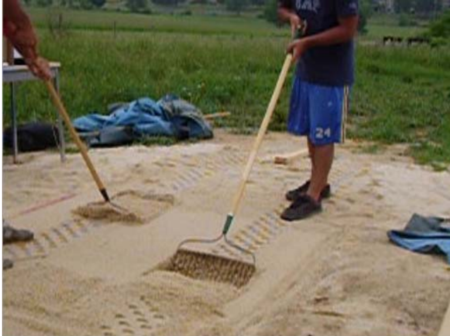
Figure 6-14: Sand Grooming Using Rakes to Remove Sand Compaction (Spring/Summer 2007)
