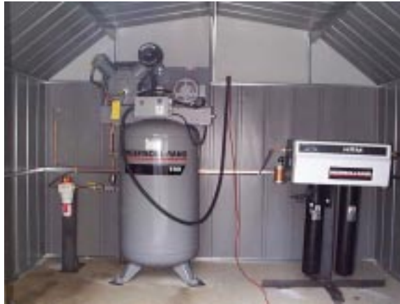
Figure 2.11: Compressor, Dryer, Filter combination
