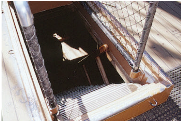
^^ Access stairs to get below deck
