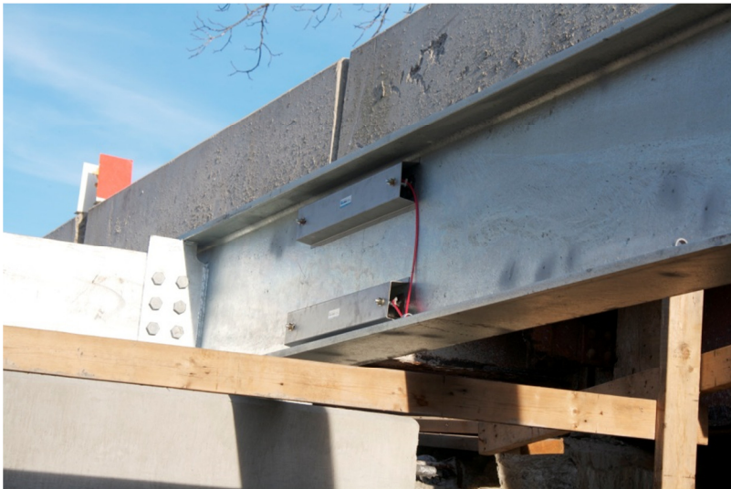
Figure 3-12. Photograph of Gauge Cover Plates on Beam C
