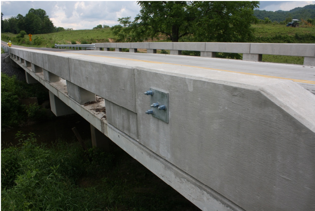
Figure 1-8. Photograph of the Completed Bridge from June 2012
