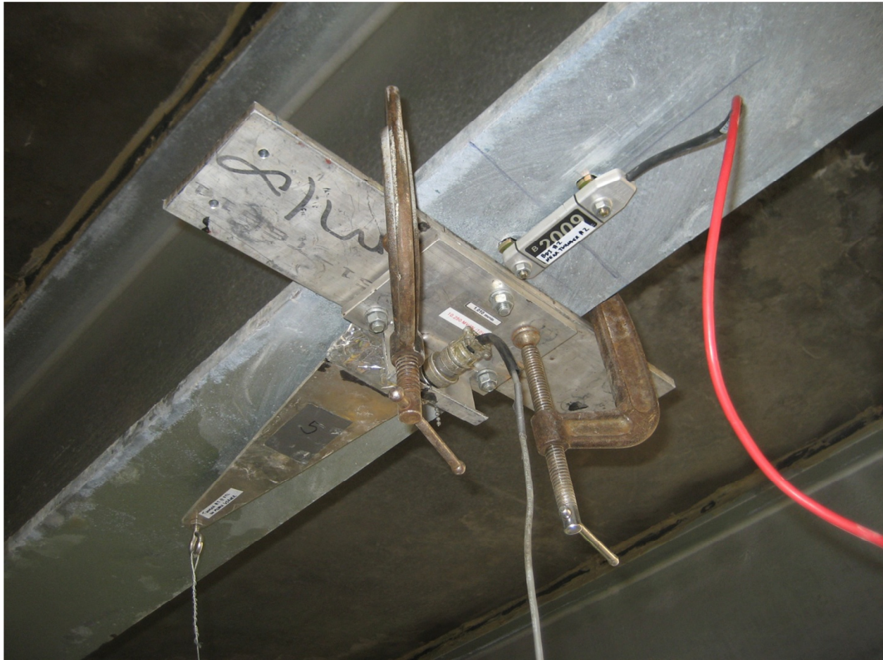
Figure 3-18. Photograph of Twanger Attached to Bottom of Girder
