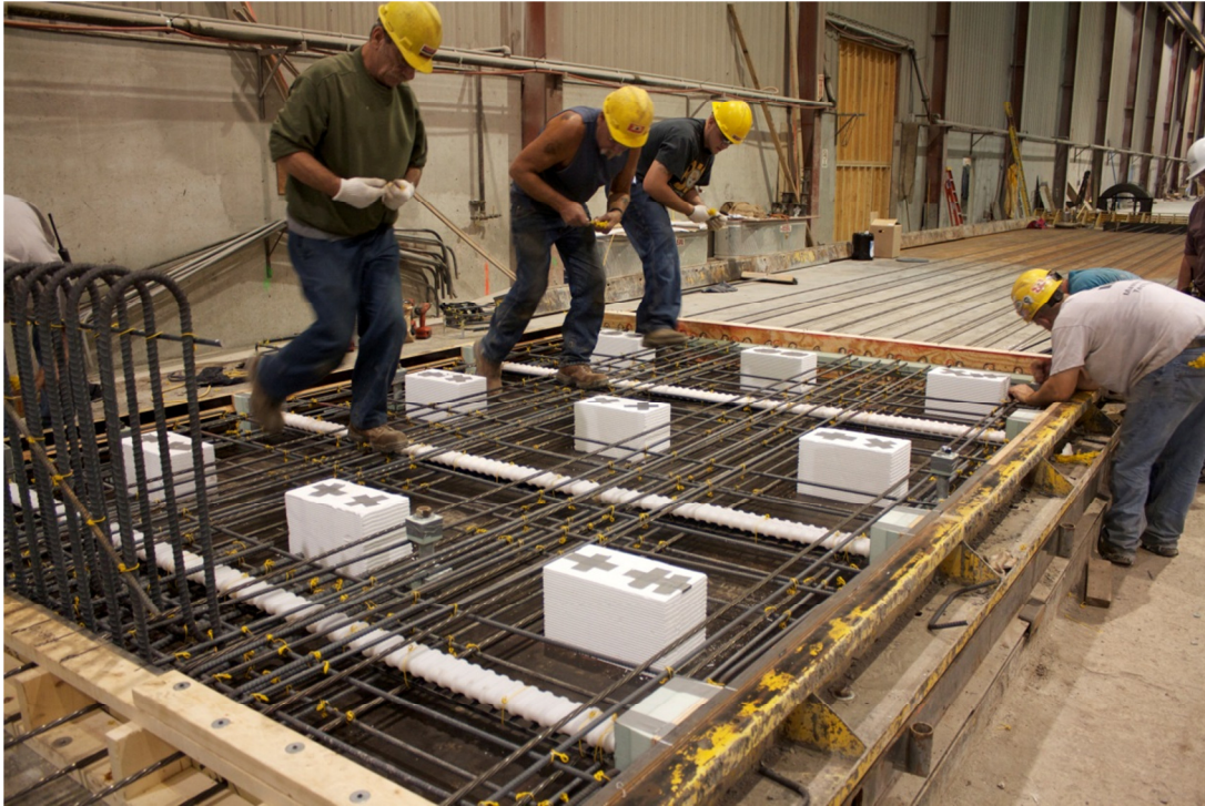
Figure 1-5. Photograph of a Deck Panel Being Constructed at Newcrete
