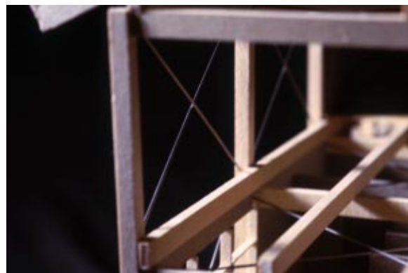
A hierarchy of girder and beam construction provides a repetition of connections, accentuating the linear nature of the building.
