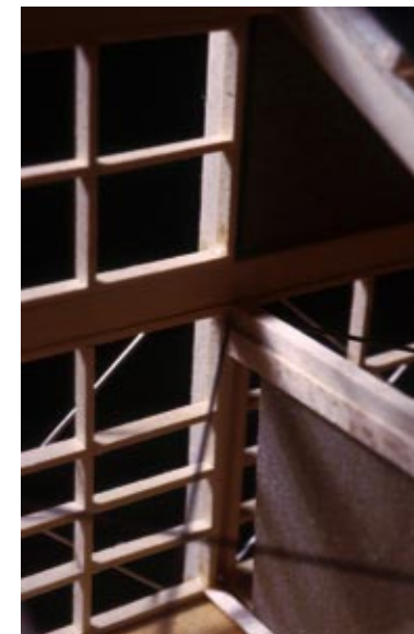
The cathedral ceiling allows the exposed connections and tension rods to invade the space without overwhelming it.
