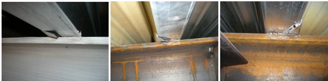
Figure 6.2: Examples of shear stud failures at the end of Static Test 2
