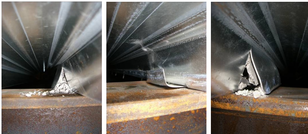
Figure 6.10: Examples of shear stud failures at the end of Static Test 3
