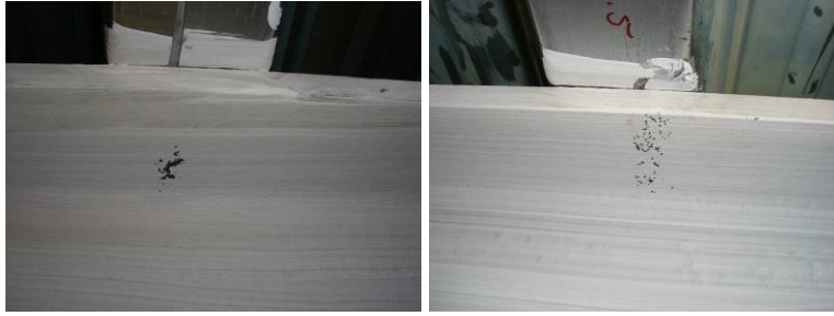
Figure 6.5: Localized top flange yielding under shear studs
