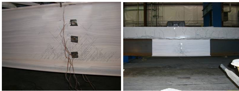
Figure 6.4: Specimen damage in girders and deck at the end of Static Test 2
