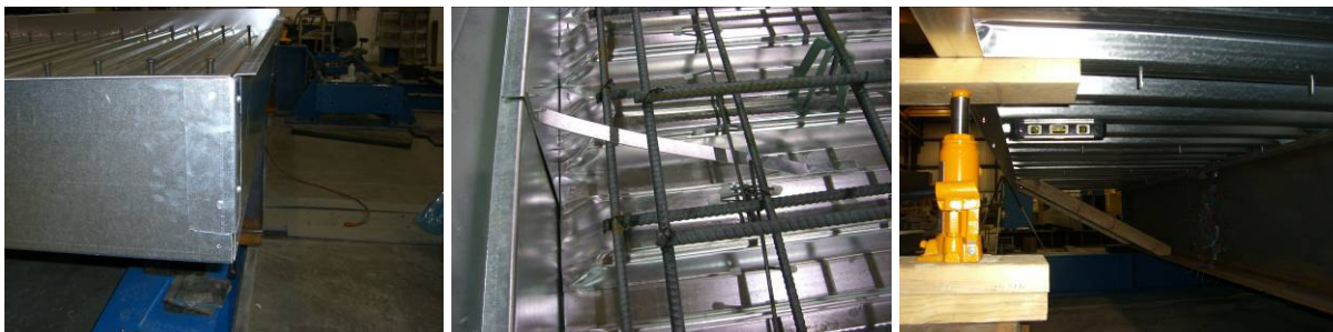
Figure 3.10: Concrete deck formwork details (a) pour stop corner (b) pour stop support straps (c) timber kickers
