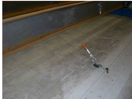
Figure 3.5: Removal of girder lateral sweep
