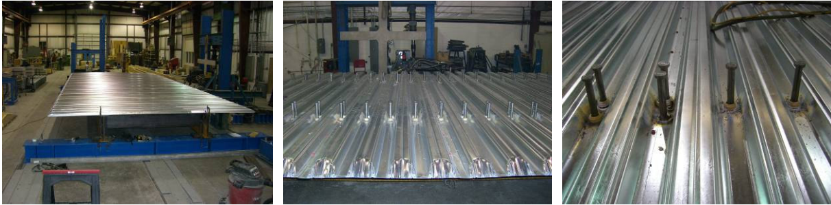
Figure 3.8: Steel deck construction details (a) at form placement (b) swedging of steel deck (c) welded shear studs
