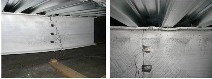
Figure 6.12: Specimen damage in steel girders at the end of Static Test 3
