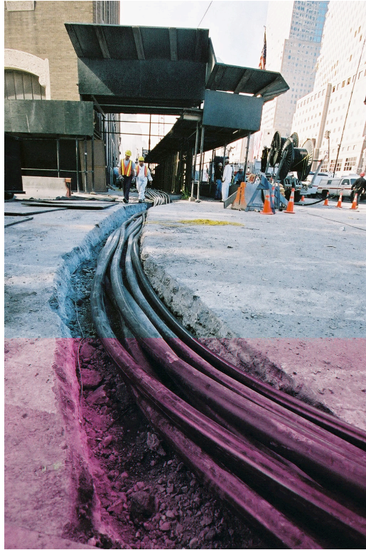
Figure 4 – Trenches dug in the street to place cables.
