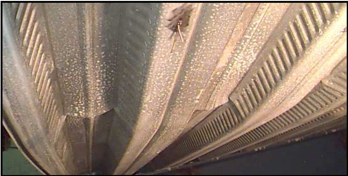
Figure 4.5.1. 4 Failed Deck for 2-0.125i-a Specimen
