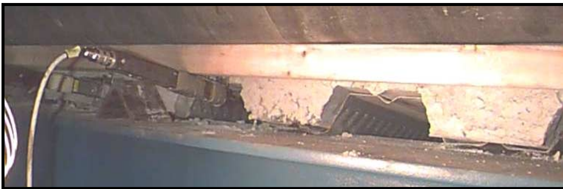
Figure 4.5. 1 End Slip of Failed Specimens
