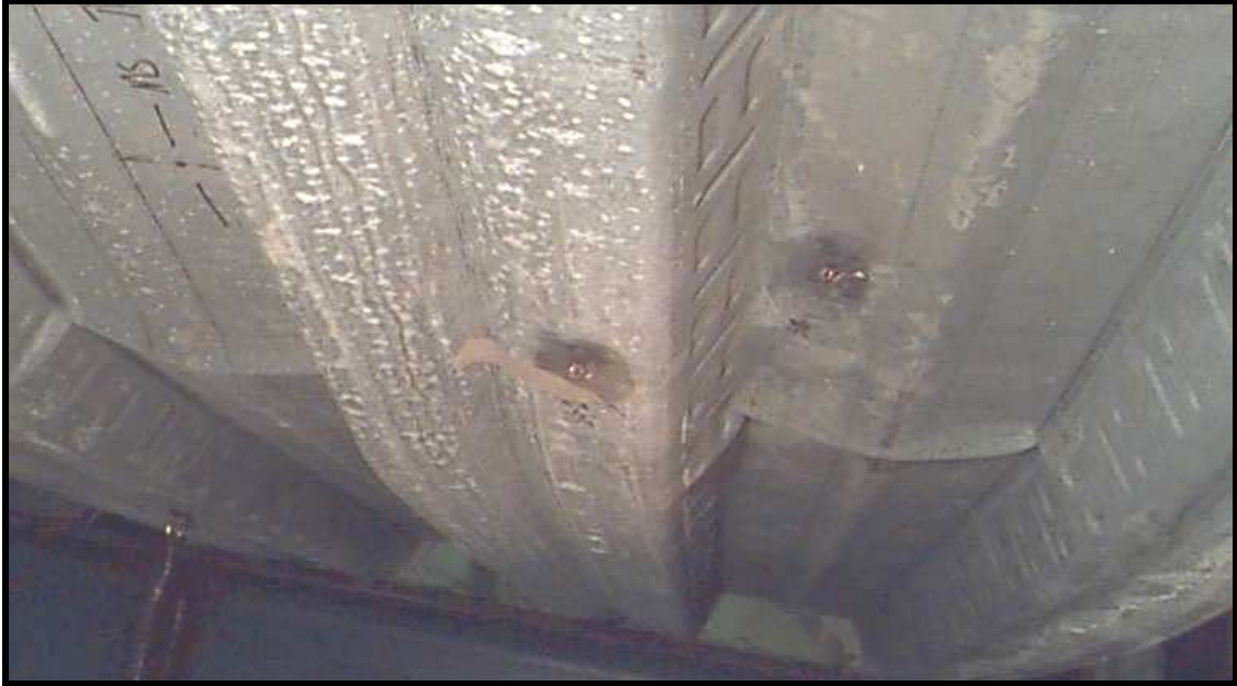
Figure 4.5.1. 3 Failed Deck for 2-exist-b Specimen
