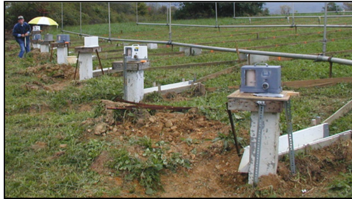
Figure 4. Installation of the FW-1 stage recorders, flumes, and stilling wells
