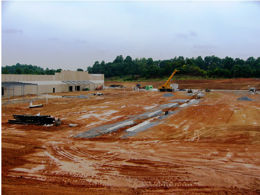
Construction of new surface lot Lynchburg, Virginia
