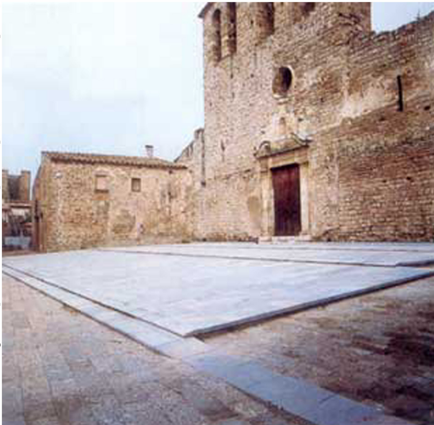
Broad step paving at building entry
