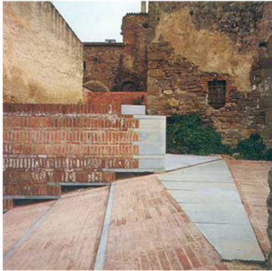
Brick and stone slab paving
