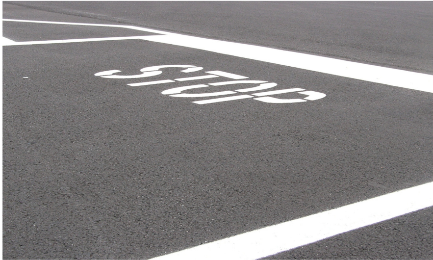
Mono-texture of new asphalt paving
