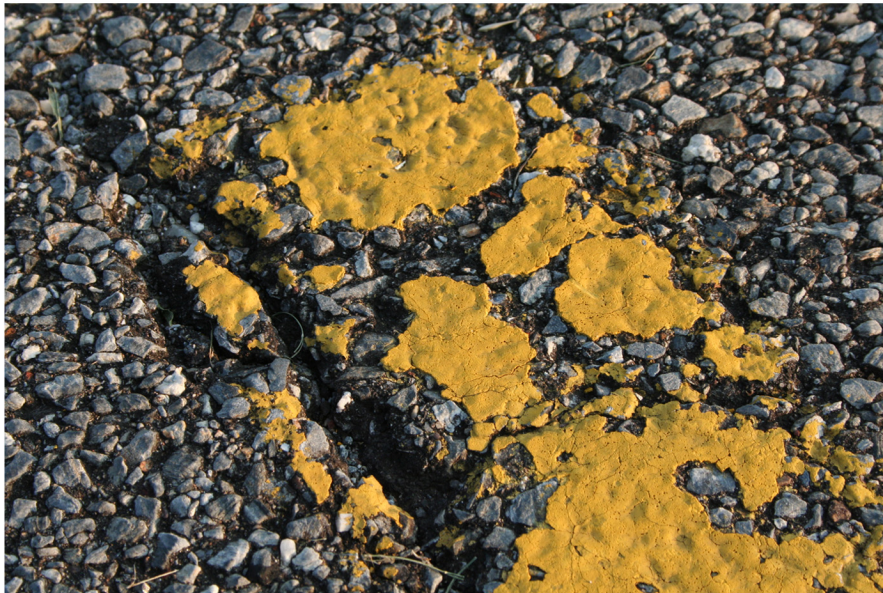
Paint stripe clinging to deteriorated asphalt
