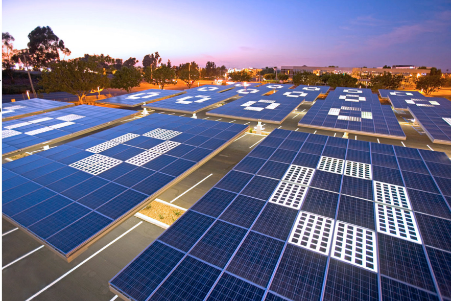
Kyocera Solar Grove Installation San Diego, California Architect: Tucker Sadler, 2005
