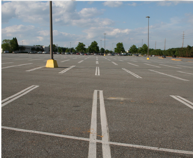
Double-striping, River Ridge Mall Lynchburg, Virginia
