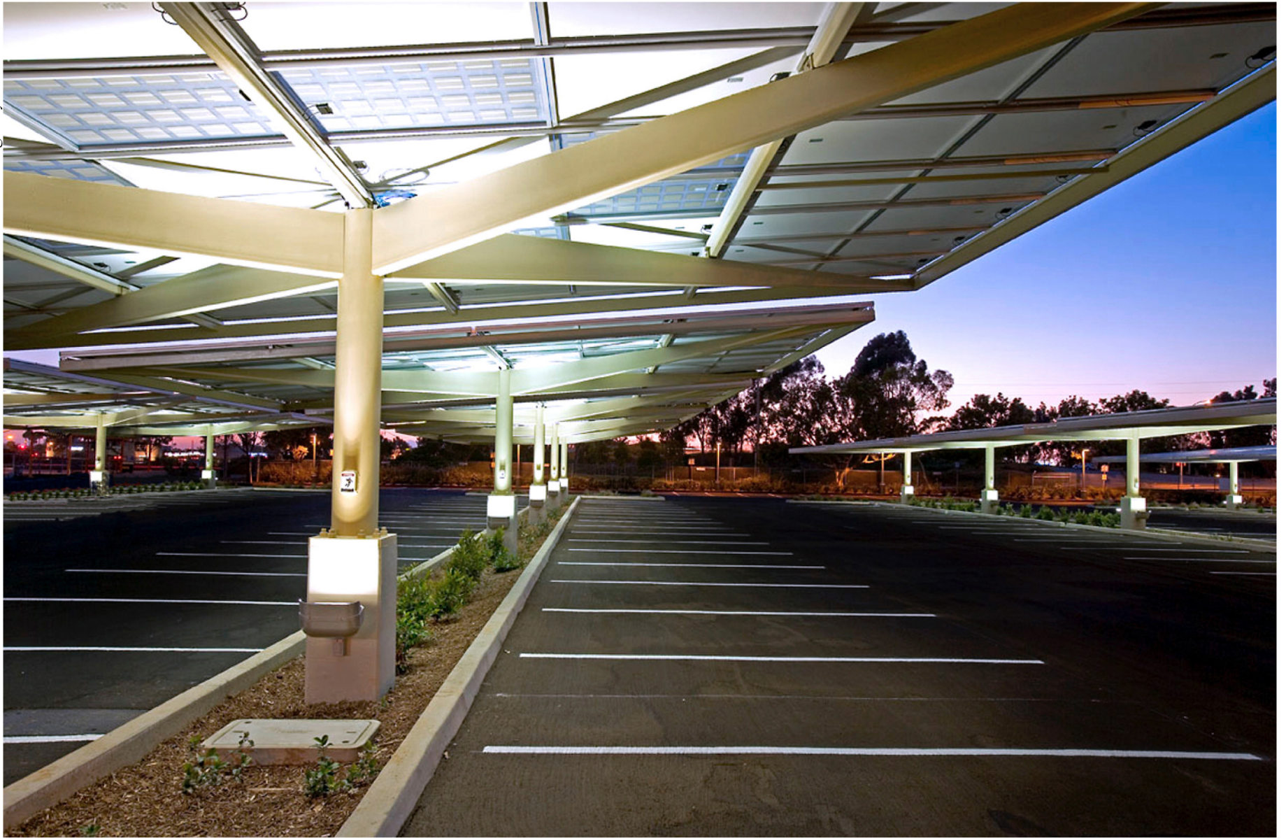
Kyocera Solar Grove Installation San Diego, California - 2005 Architect: Tucker Sadler
