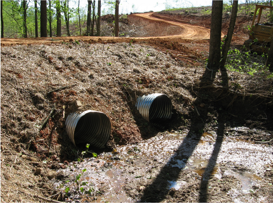
Figure 5. Typical corrugated steel culverts used as a stream crossing.
