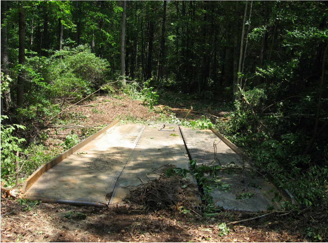
Figure 2. Typical 3-panel steel skidder bridge.
