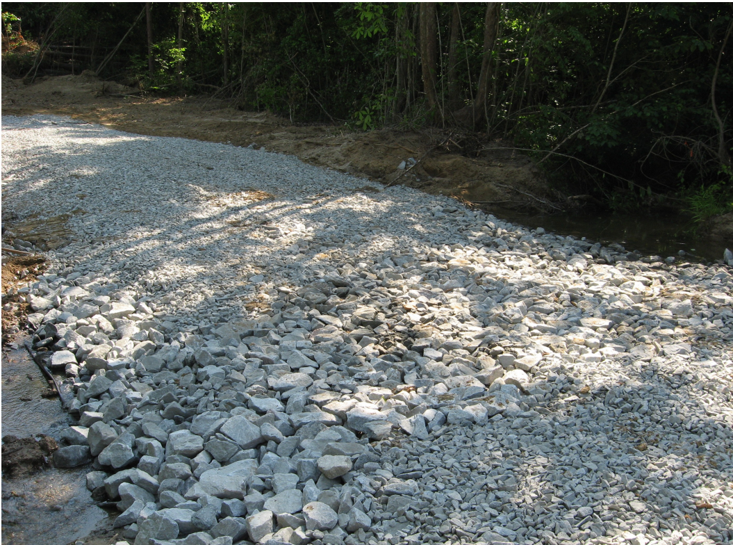
Figure 4. Typical ford crossing re-enforced with geotextile and stone.
