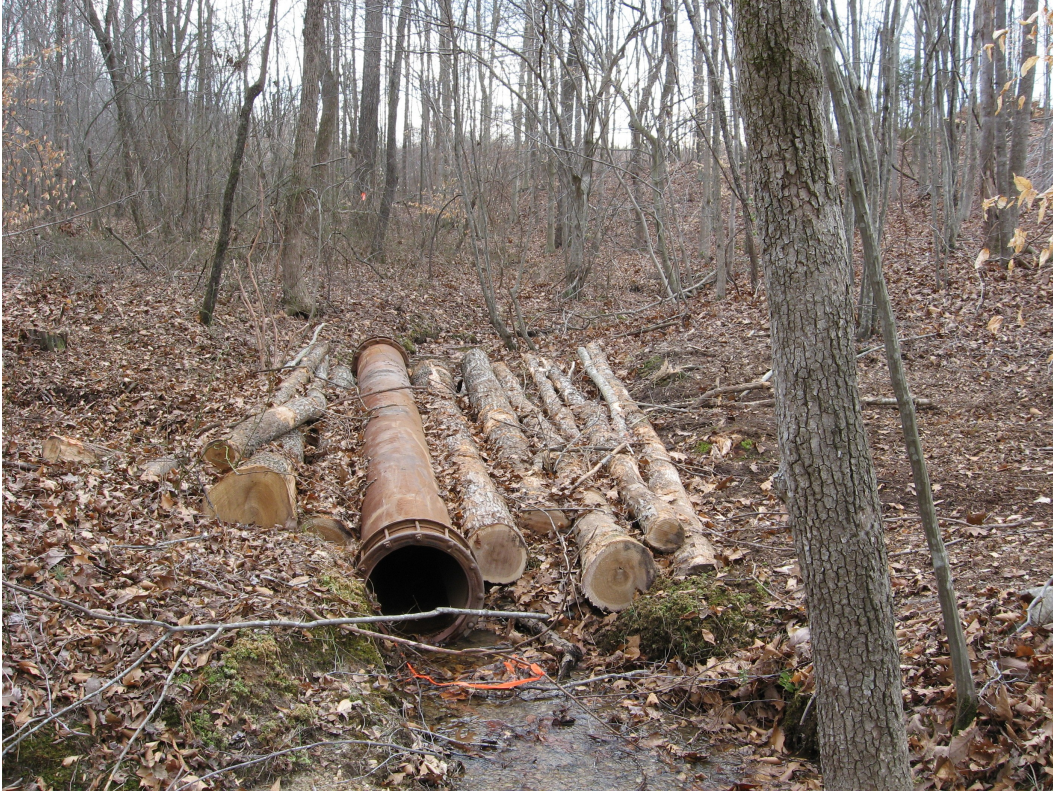
Figure 38. Pole bridge installed with pipe and white oak poles in an intermittent stream.
