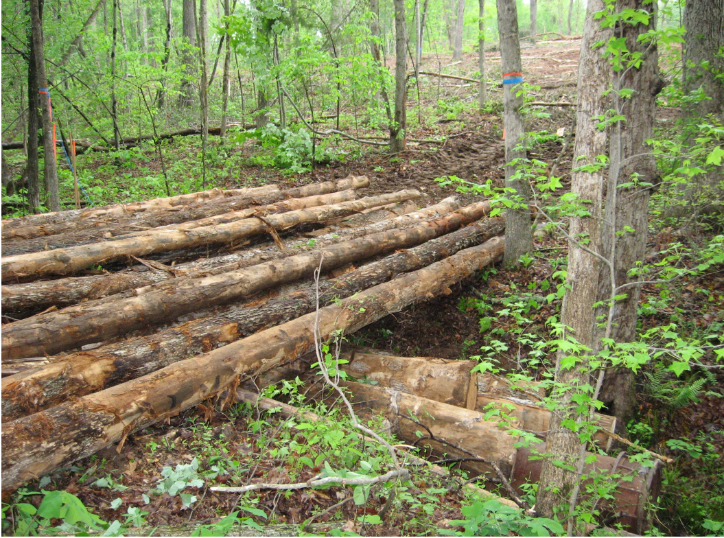
Figure 3. Pole bridge constructed with a steel pipe and white oak logs both parallel and perpendicular to stream channel.
