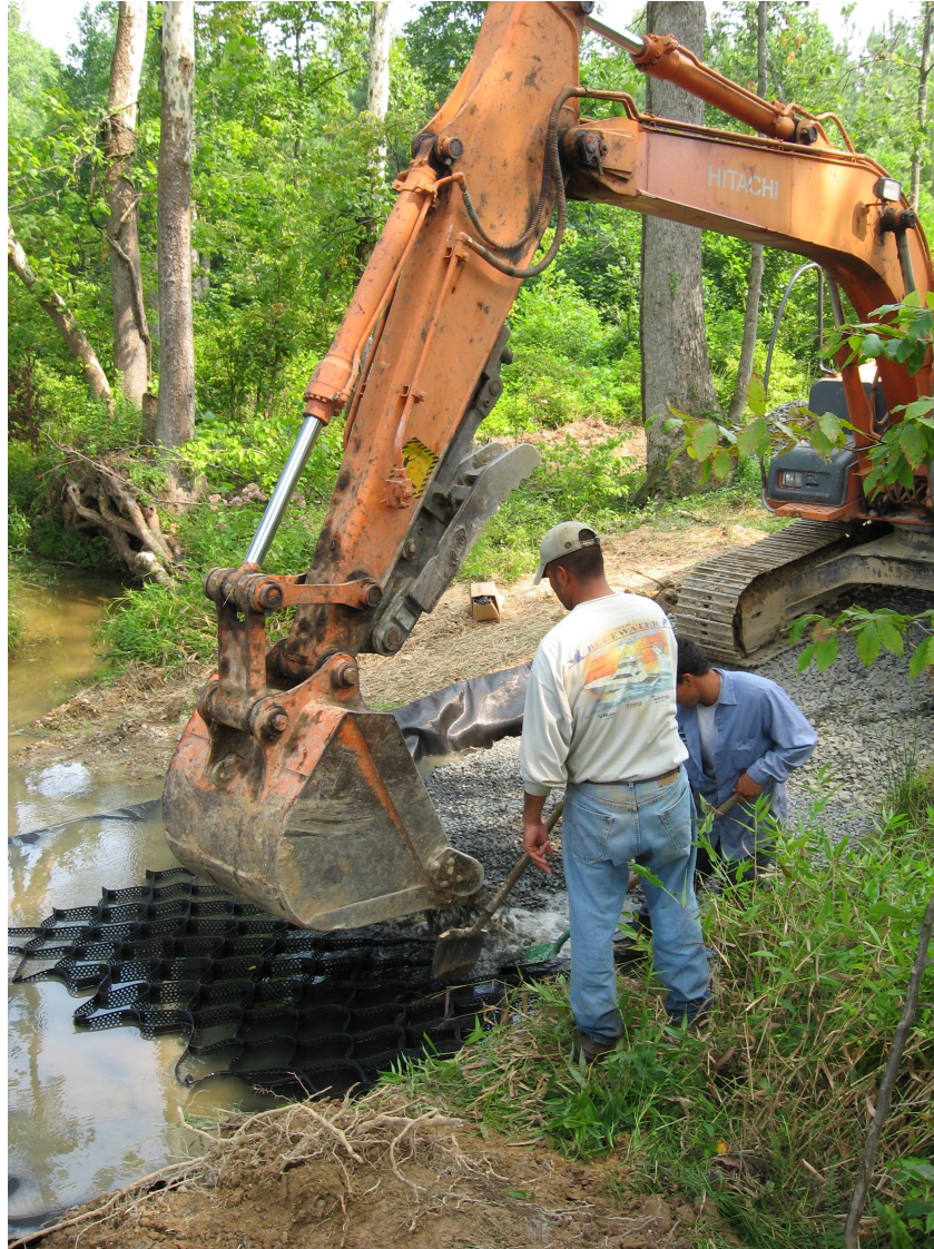
Figure 37. Applying limestone gravel (size #57) to a ford re-enforced with GeoWeb and geotextile.
