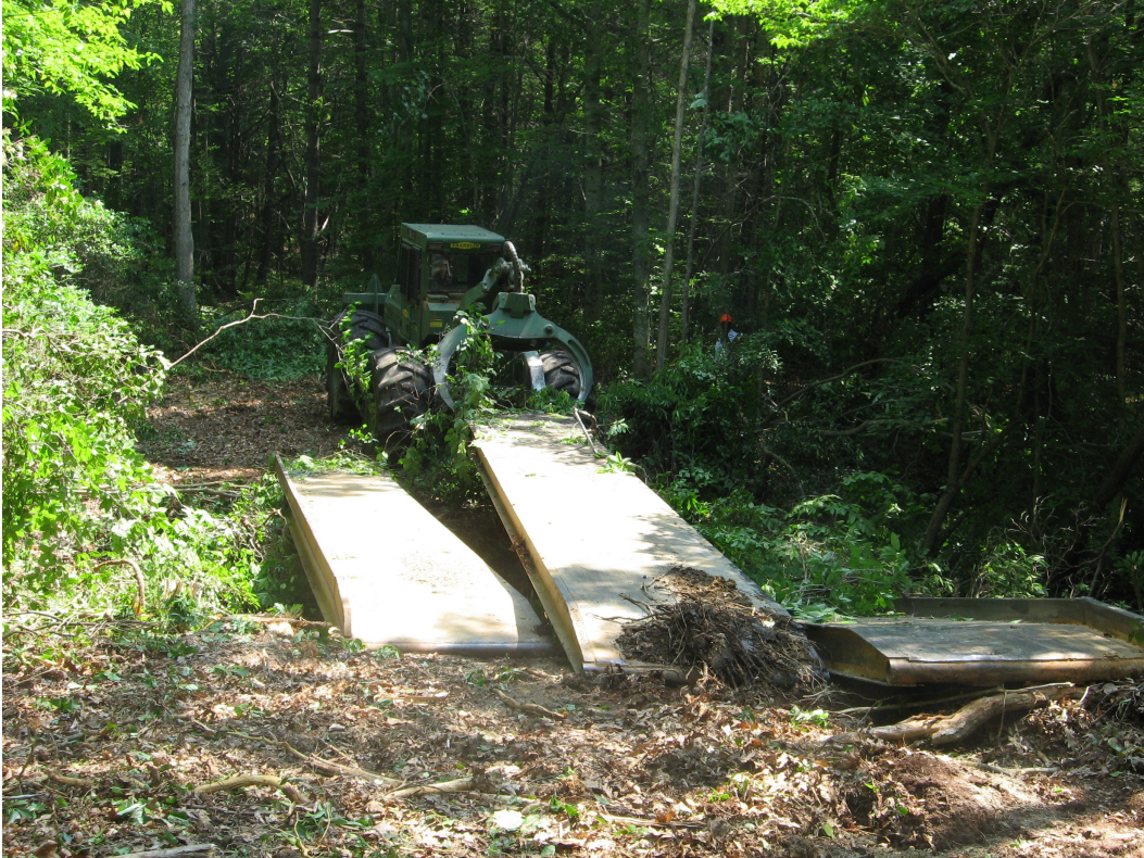
Figure 35. Steel bridge installation by a skidder. This particular set of bridges is 40 feet long and consists of three panels.
