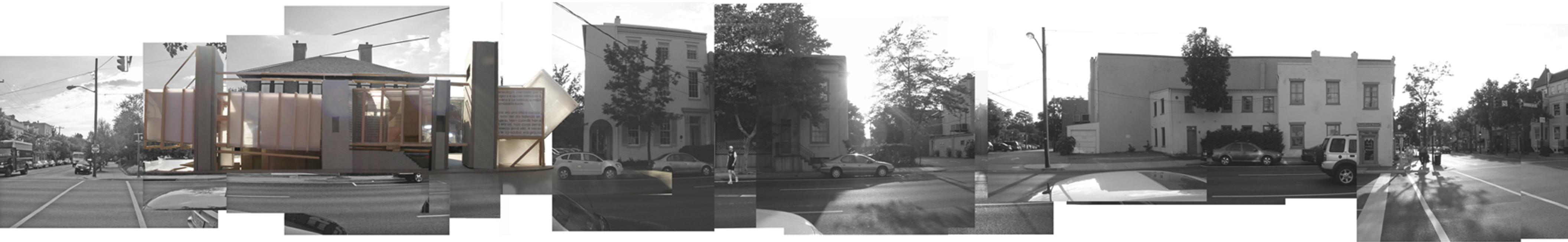
elevation on South Patrick St /between Prince st. and King st./
