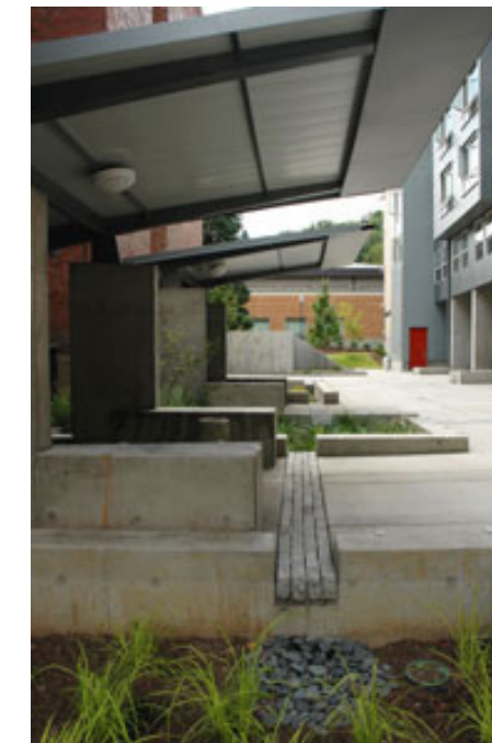
Figure 3.25: View of the rainwater collection system
