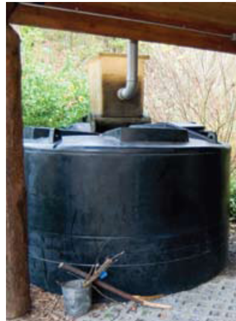
Figure 3.31: View of the rainwater storage cistern (Source: www.seattle.gov , 2011)
