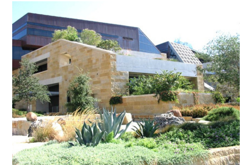
Figure 2.18: View of green roof (Source: www.greenroofs.com , 2011)
