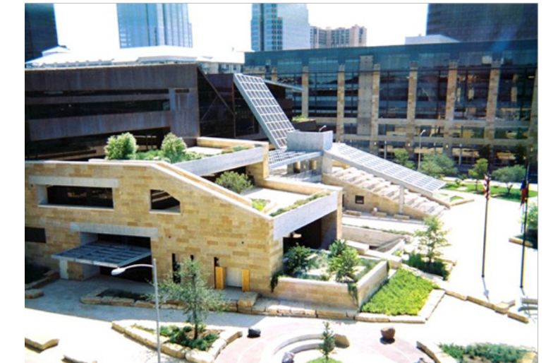
Figure 2.17: View of Green roof (Source: www.greenroofs.com , 2011)
