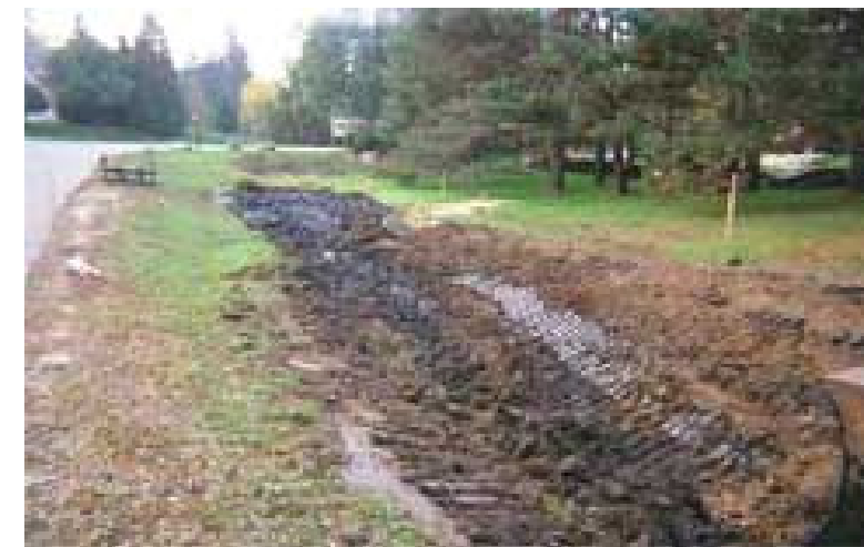
Figure 4.16: Existing drainage ditch at Meadowlake farms prior to construction (Source: Niswander Environmental, 2005)
