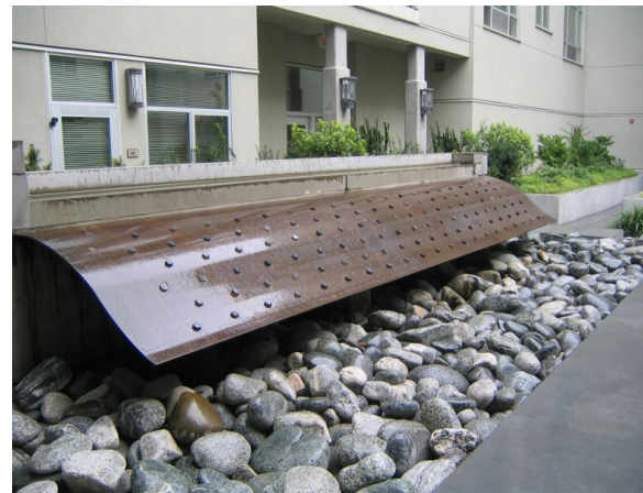
Figure 3.18.2: View of Cor-ten steel plates with multi colored glass buttons
