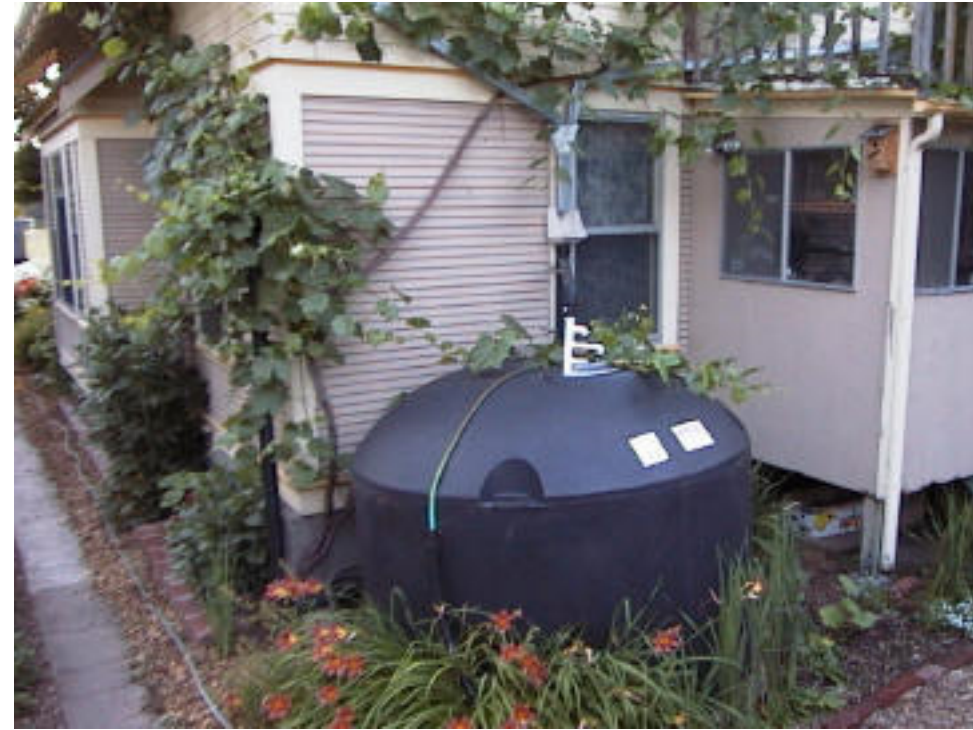
Figure 3.1: Residential rainwater harvesting system (Source: www.rwh.in , 2011)
