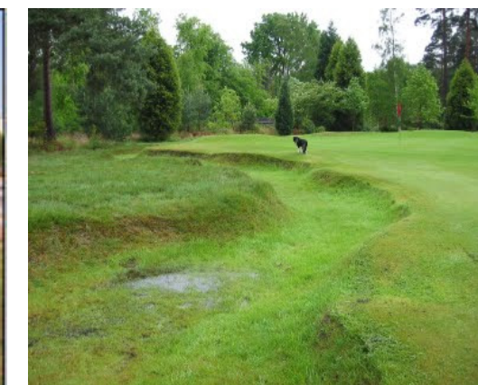
Figure 4.5: Wet swale (Source: www.golfcoursetravelblog.blogspot.com , 2011)
