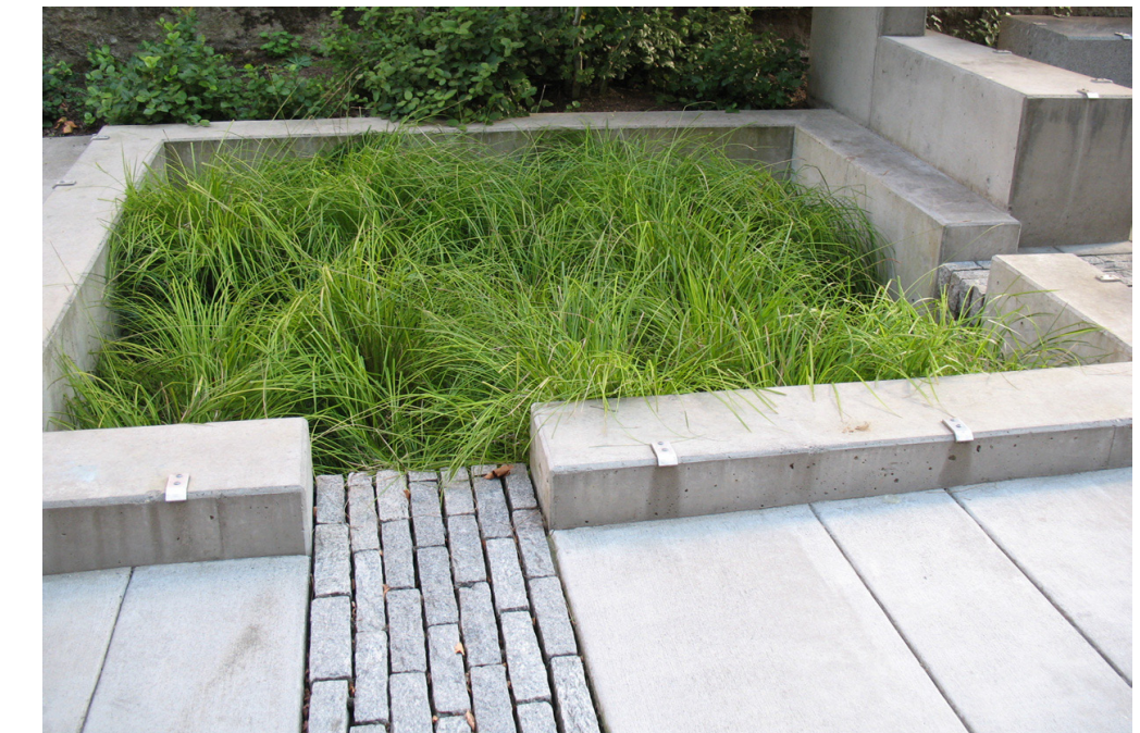
Figure 3.26: View of the rainwater collection splash box
