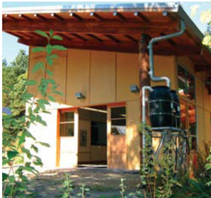
Figure 3.30: View of the Rainwater harvesting system (Source: www.seattle.gov , 2011)
