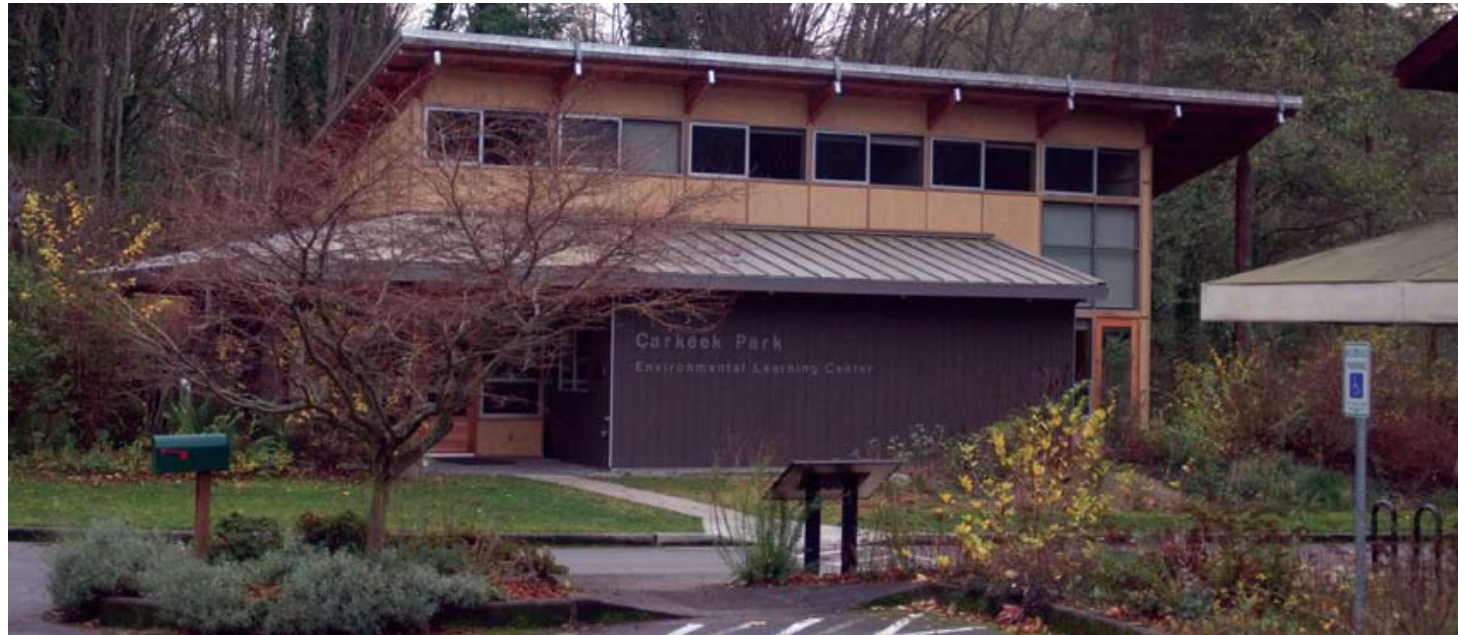
Figure 3.27: View of the Environmental Learning Center (Source: www.seattle.gov, 2011)
