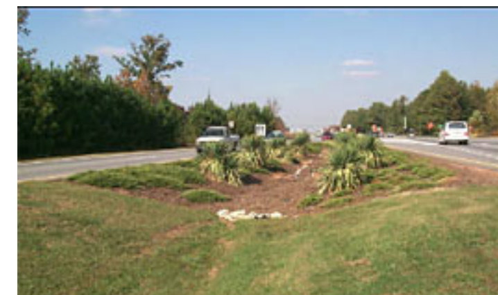
Figure 4.4: Dry Swale (Source: www.tvaed.com/sustainable , 2011)
