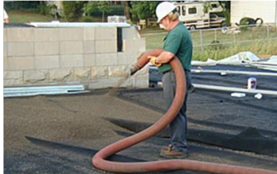
Figure 2.36: Installing drainage course using pneumatic media handling methods
