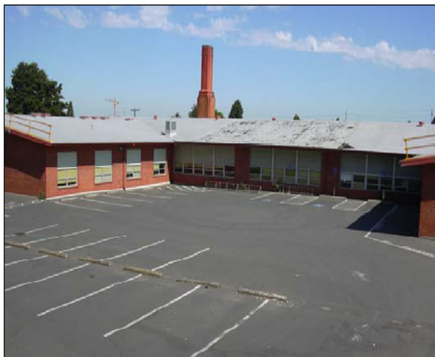
Figure 4.14: Prior to construction, looking north across the parking lot toward the site of the rain garden. The parking swale was constructed between rows of parking stalls in the foreground. (Source: Portland Bureau of Environmental Services, 2004)
