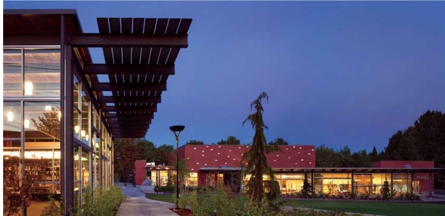
Figure 3.23: View of Northgate Civic Center (Source: www.seattle.gov , 2011)
