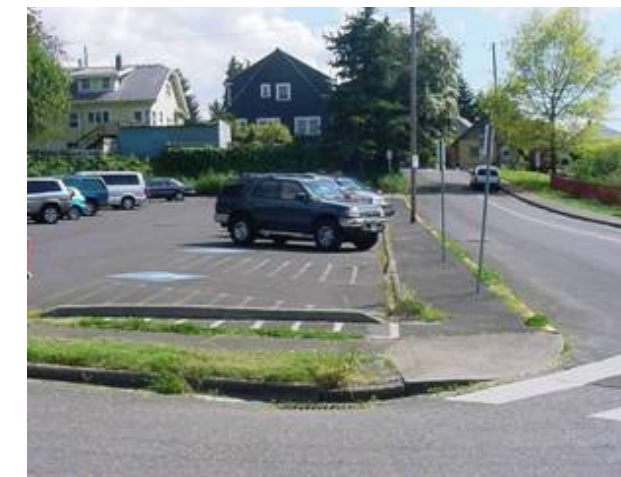
Figure 4.7: View of Glencoe Parking Lot before retrofit (Source: Portland Bureau of Environmental Services, 2004)
