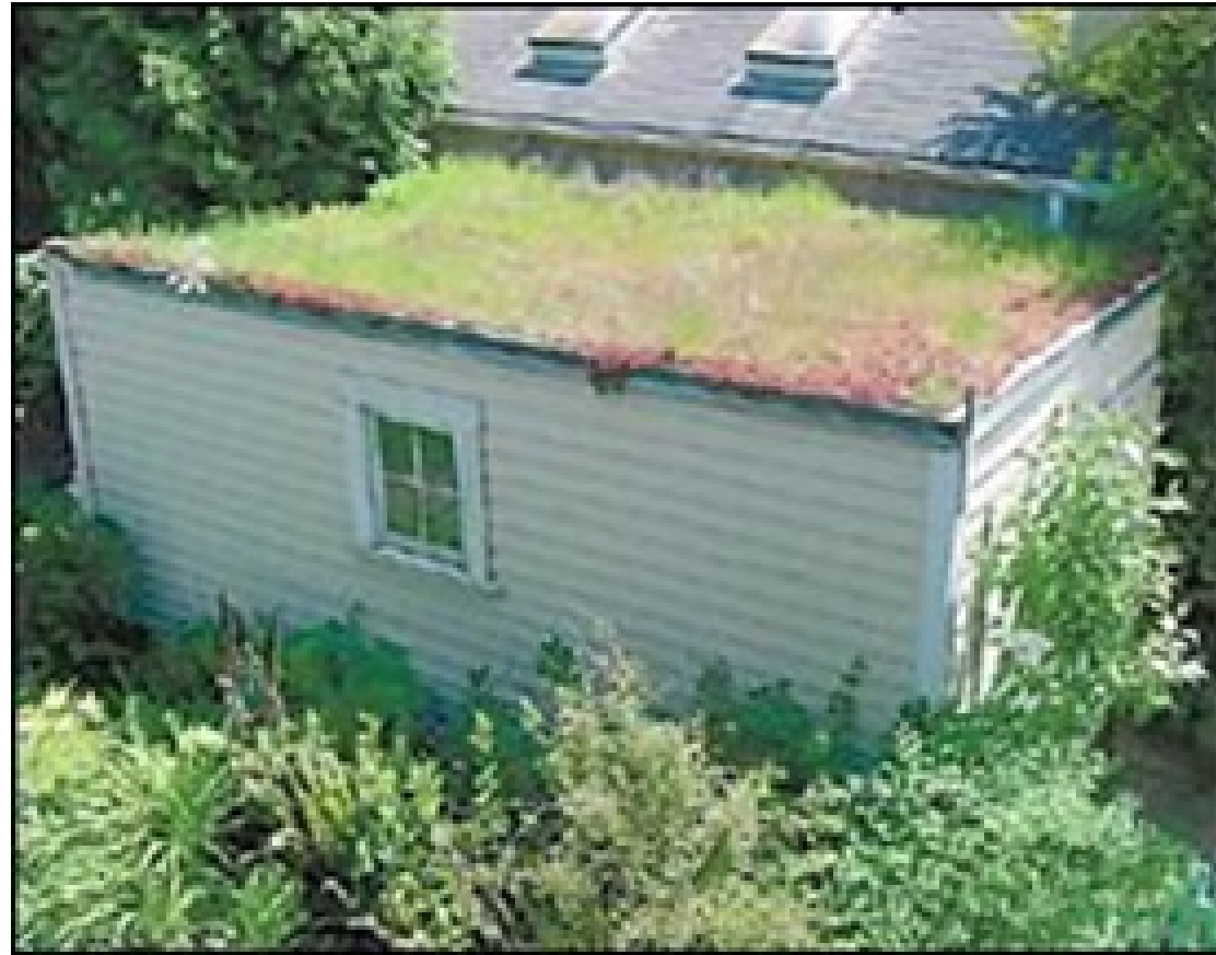
Figure 2.14: View of the green roof on Liptan Garage, Portland (Source: www.landscapeandurbanism.blogspot.com , 2011)
