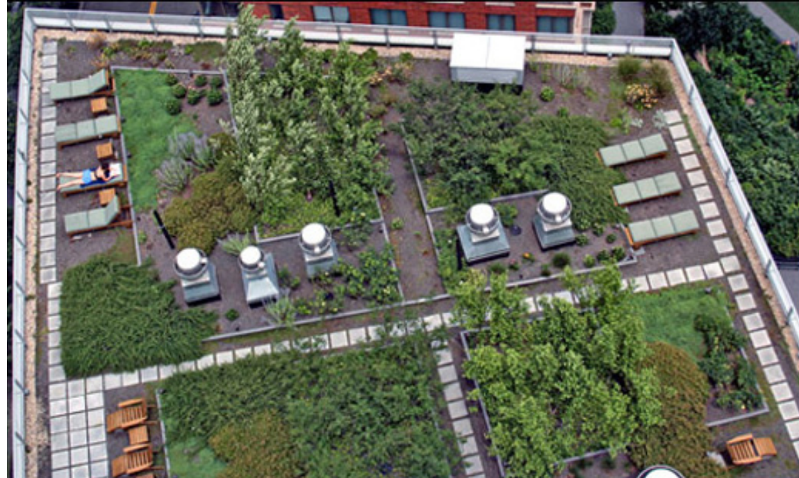
Figure 2.11: View of the green roof on Solaire, New York (Source: www.streetsblog.org)2011
