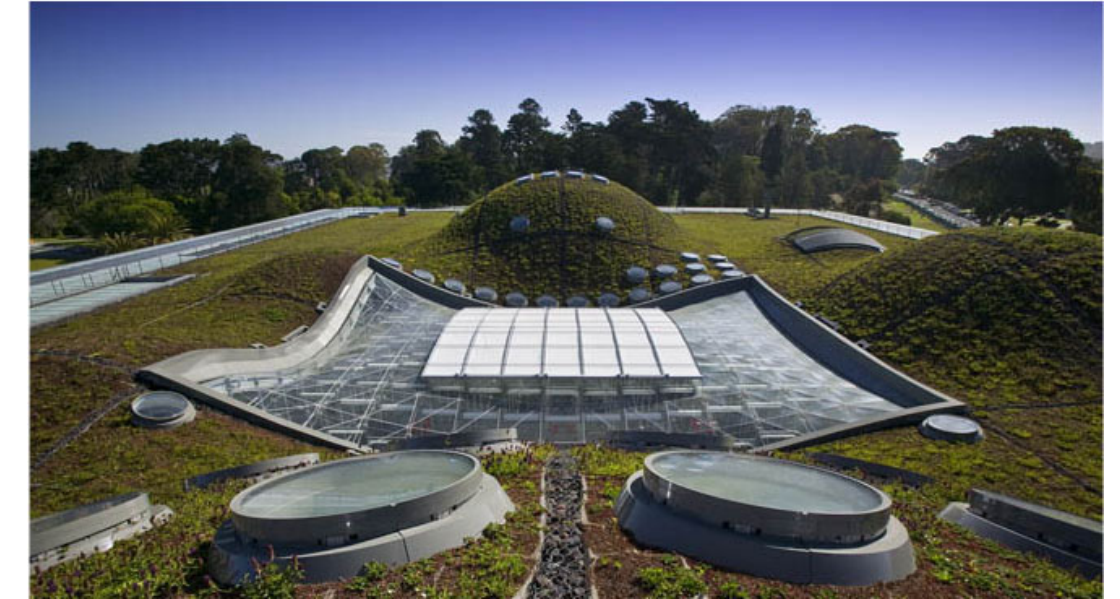
Figure 2.33: Natural lighting system in the green roof system (Source: www.archdaily.com, 2011)
