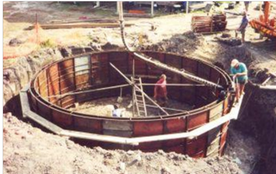
Figure 3.12: Cast in-situ, below ground storage tank (Source: www.rainharvesting.com.au/concrete_tanks.asp , 2011)
