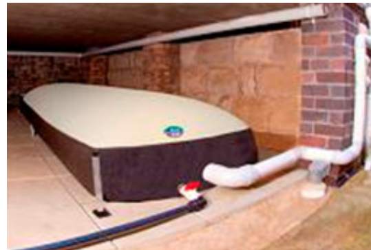
Figure 3.16: Bladders, used as sub-floor or underground storage (Source: www.rainharvesting.com.au , 2011)
