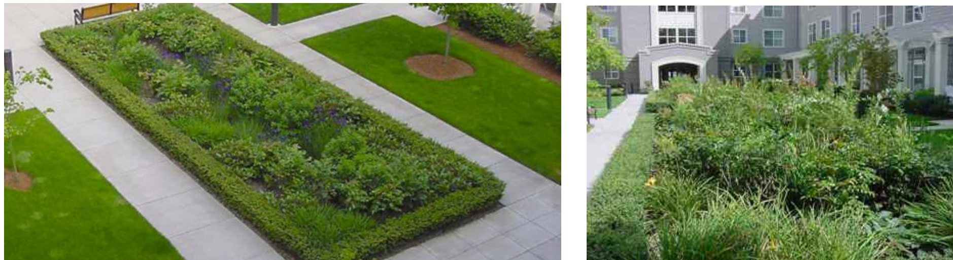
Figure 5.1: Buckman Heights courtyard infiltration basin (430 NE 16th Ave)
