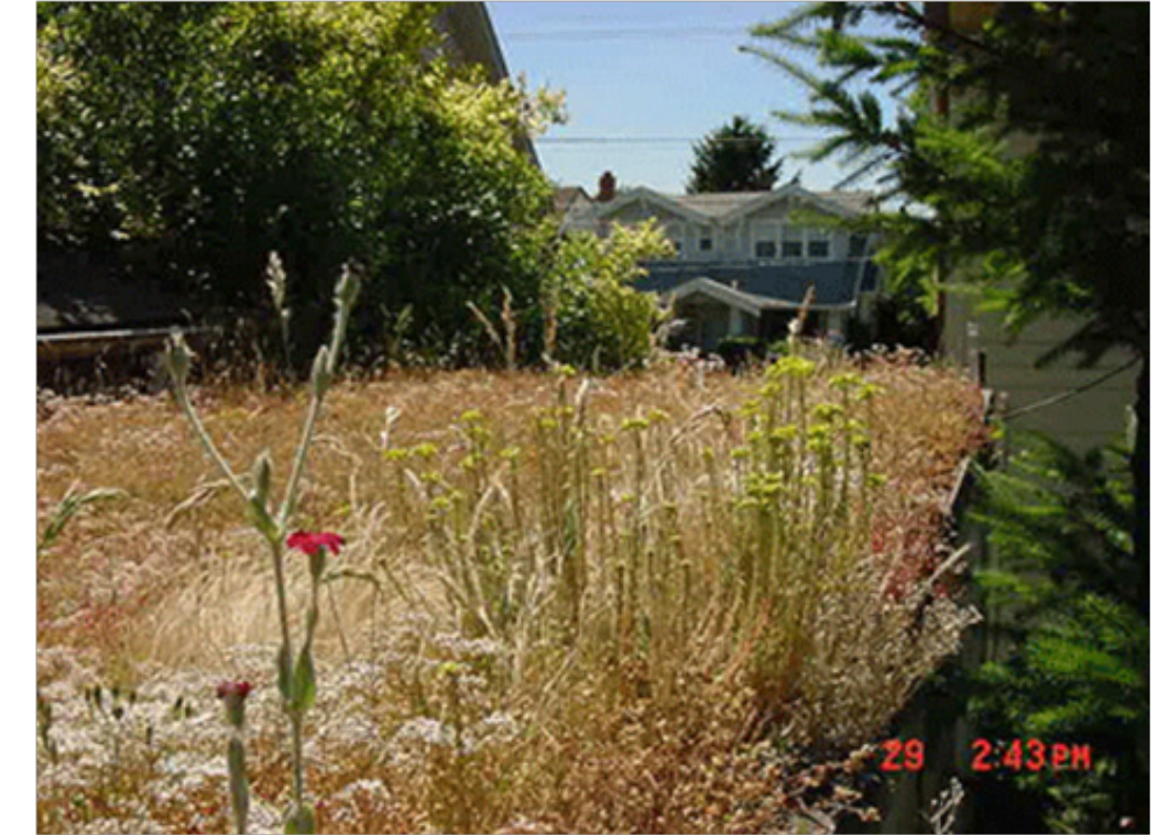
Figure 2.15: View of vegetation on the green roof (Source: www.greenroofs.com , 2011)
