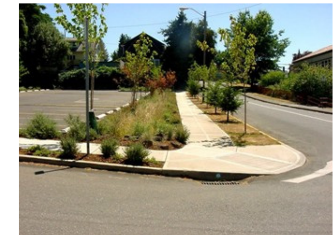
Figure 4.8: View of Glencoe Parking Lot after retrofit (Source: Portland Bureau of Environmental Services, 2004)
