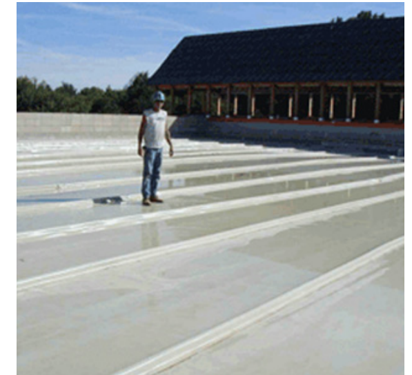
Figure 2.39: Installing innovative ponding ridges and trickle irrigation system
