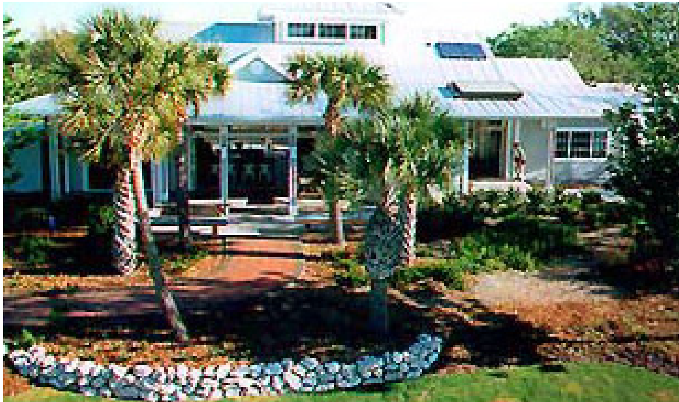
Figure 3.20: View of the entrance of the Florida Learning Center
