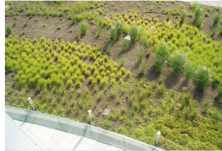
Figure 2.26: View of the natural grass vegetation on the green roof (Source: www.hydrotechusa.com, 2011)
