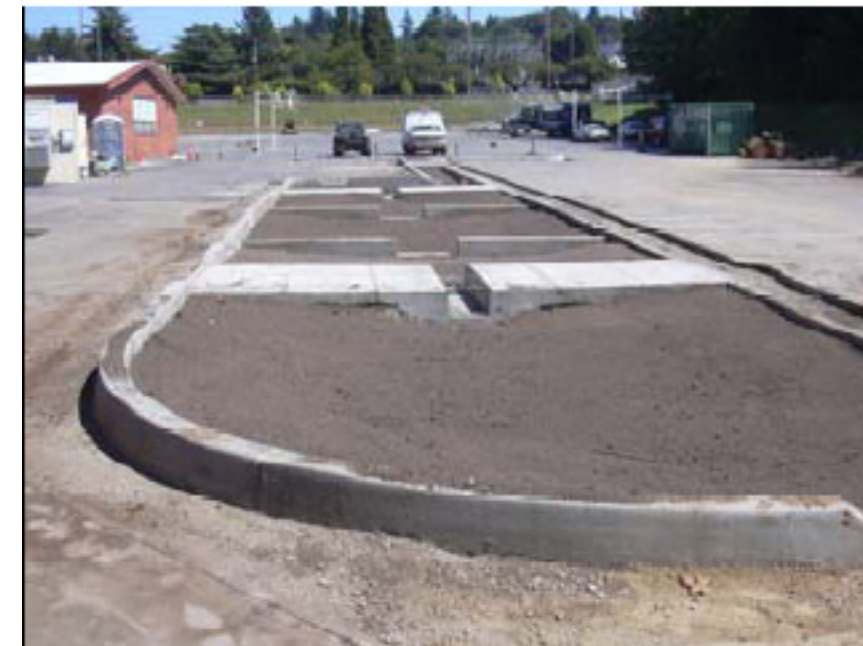
Figure 4.11: The parking lot swale after placement of 10" of imported soil, foot compaction and final grading (Source: Portland Bureau of Environmental Services, 2004)
