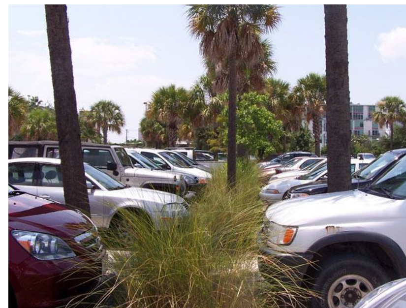
Figure 4.25: The Florida Aquarium Parking lot vegetated swale (Source: Initiative, T. S. S2008)
