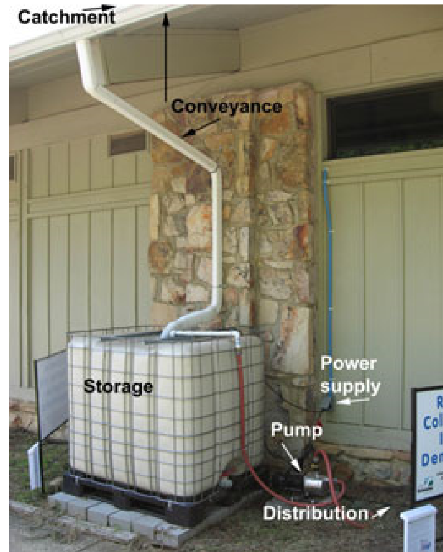
Figure 3.6: Rainwater conveyance pipes (Source: www.rainharvesting.com , 2011)
