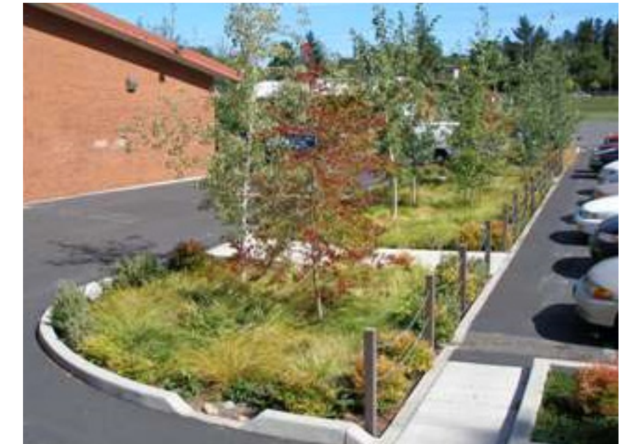
Figure 4.12: Parking lot swale after construction highlighting the curb cuts for runoff entry (Source: Portland Bureau of Environmental Services, 2004)
