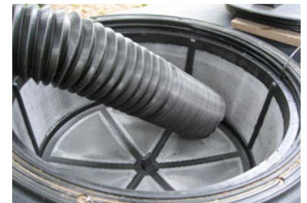
Figure 3.11: A screened basket in the manhole will prevent a lot of organic matter and mosquitoes from entering the tank. (Source: www.rainharvesting.com, 2011)
