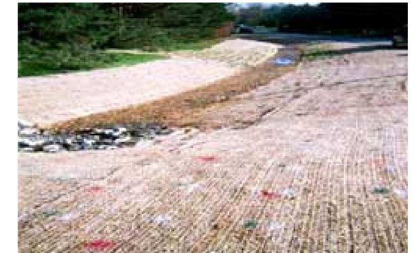
Figure 4.17: Mulch blankets used over top soil used to reduce soil erosion and stabilize new plant material (Source: Niswander Environmental, 2005)
