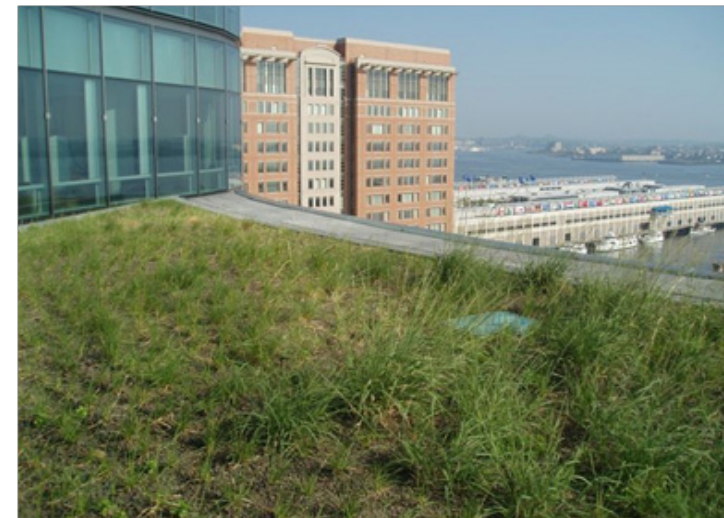
Figure 2.27: View of the natural grass vegetation on the green roof (Source: www.hydrotechusa.com, 2011)
