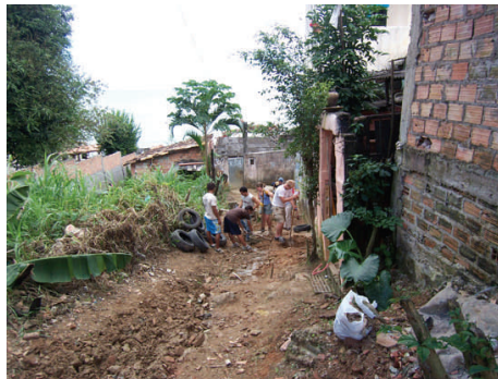
Cleaning the site - image 13
