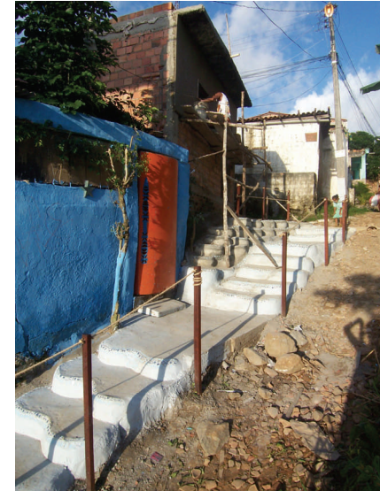
Finished stairs - image 17
