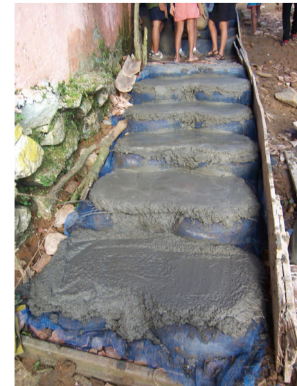
Pouring concrete - image 16
