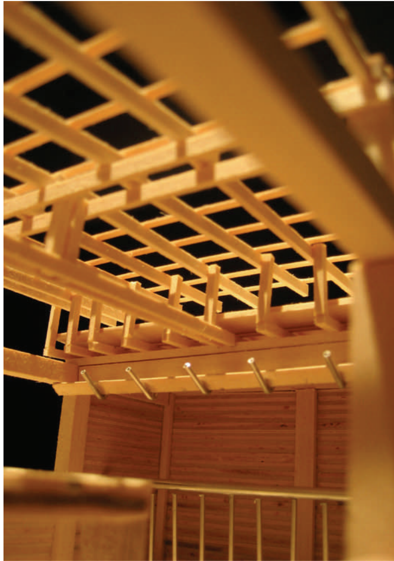
Final model temple view of roof framing
